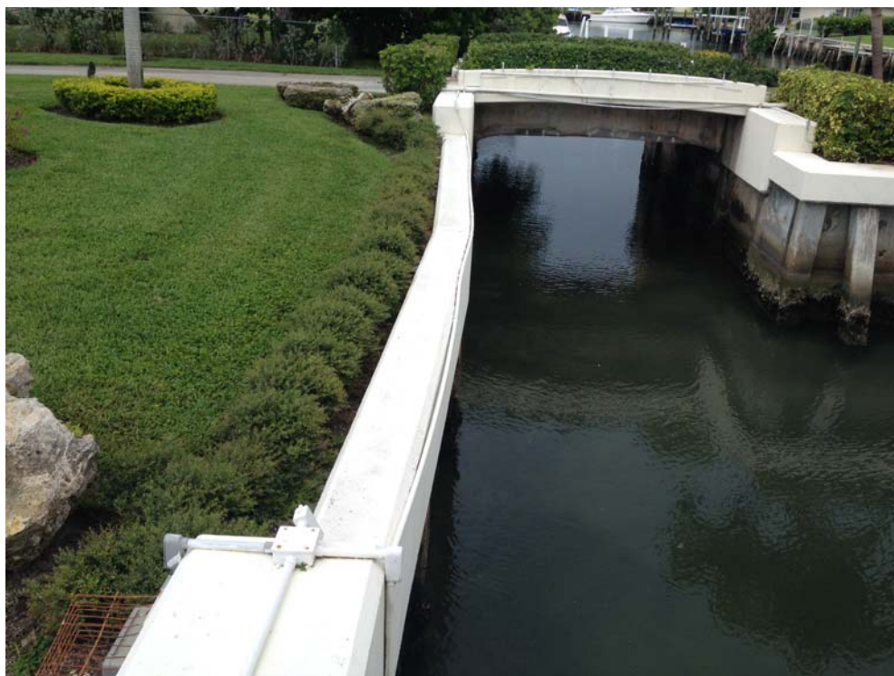
Figure 33: Bulkhead Wall Deflection Island Drive Structures
