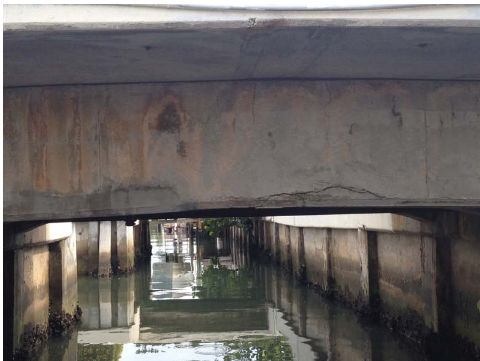
Figure 23: Beam Cracking Island Drive Structure
