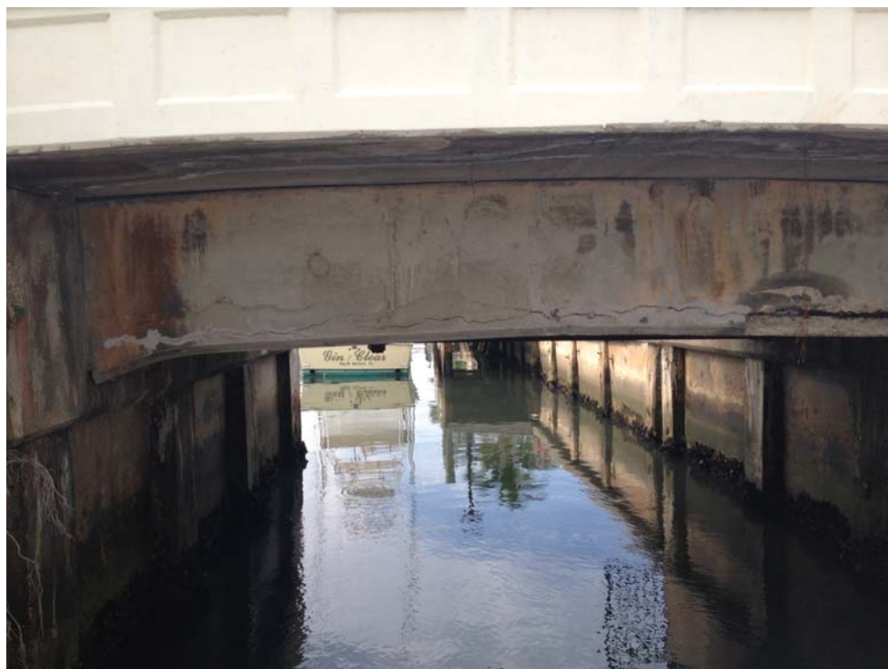
Figure 27: Concrete Spall & Beam Cracking Island Drive Structure
