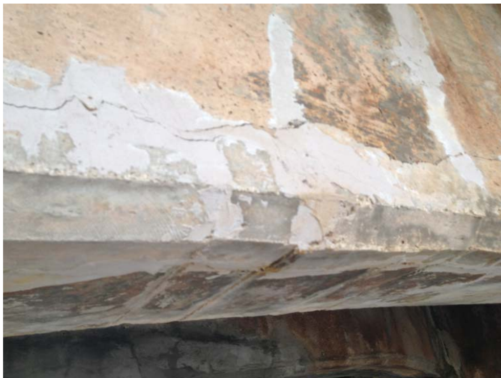
Figure 22: Beam Cracking Island Drive Structure
