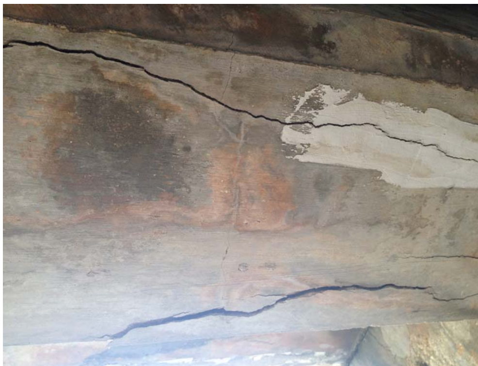
Figure 21: Beam Cracking Island Drive Structure
