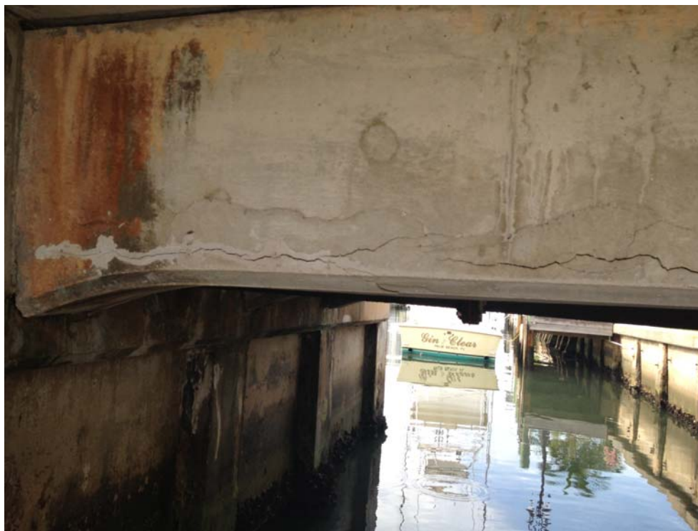
Figure 30: Beam Cracking Island Drive Structure
