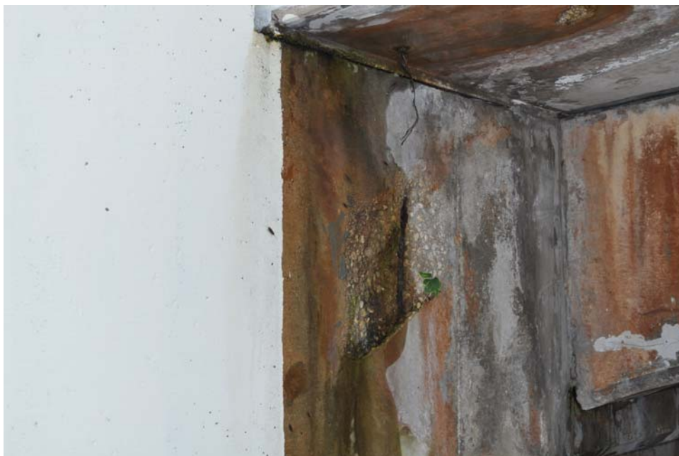
Figure 14: Cap Spall Island Drive Structure
