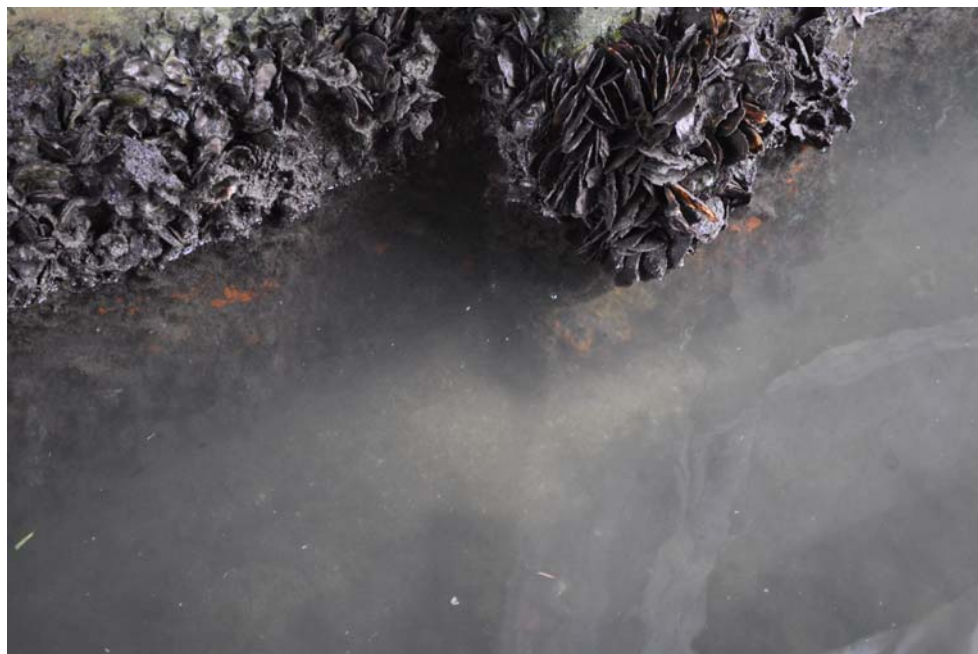
Figure 32: Retained Material Leak Island Drive Structure
