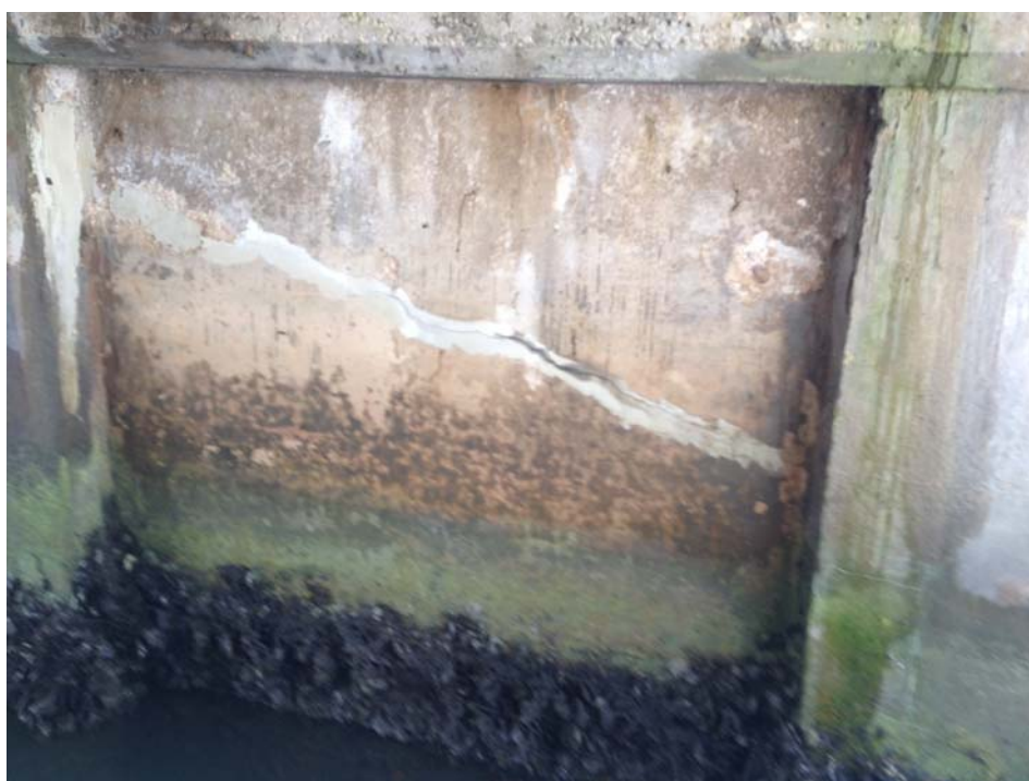
Figure 13: Sheet Panel Cracking Island Drive Structure
