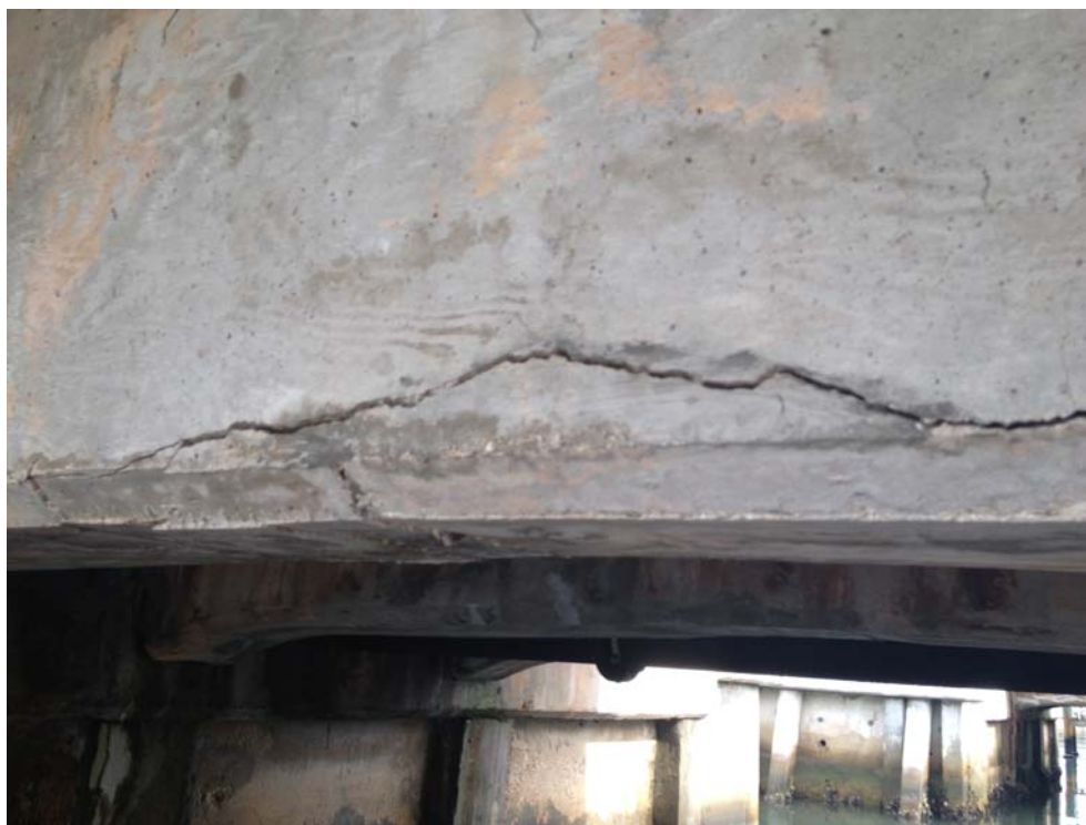
Figure 25: Beam Cracking Island Drive Structure
