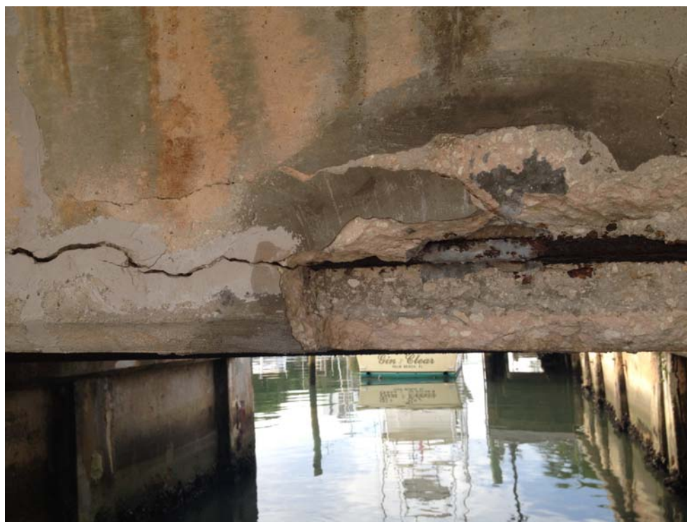
Figure 28: Concrete Spall & Reinforcing Corrosion Island Drive Structure
