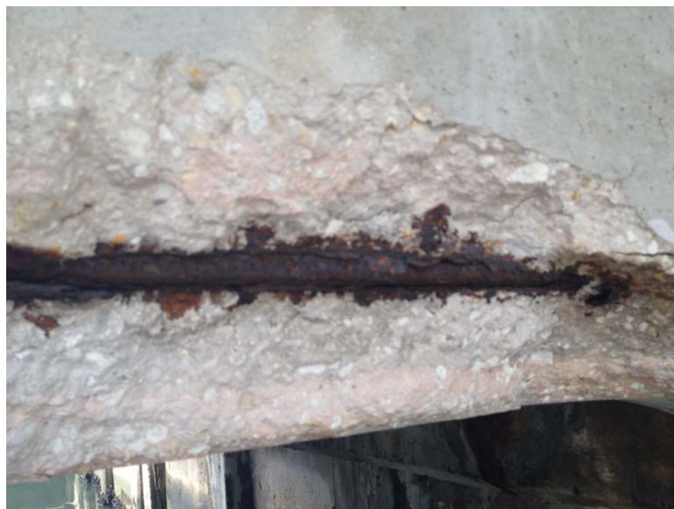
Figure 29: Reinforcing Corrosion Island Drive Structure
