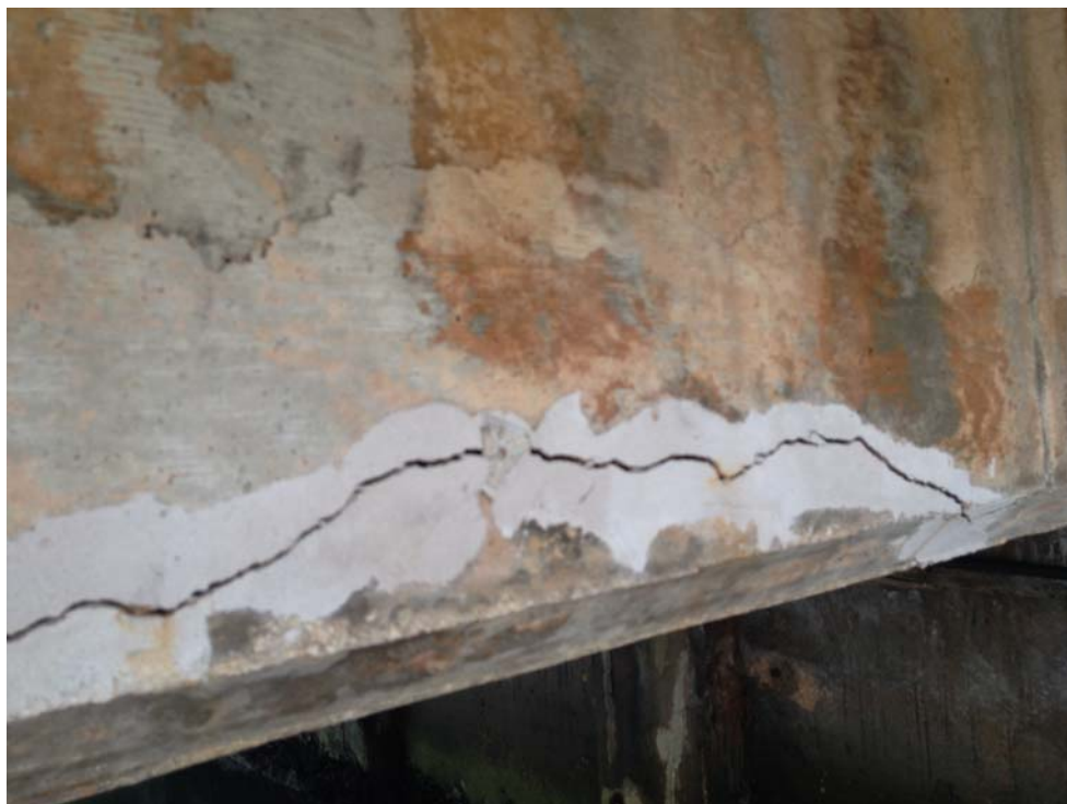
Figure 26: Beam Cracking Island Drive Structure
