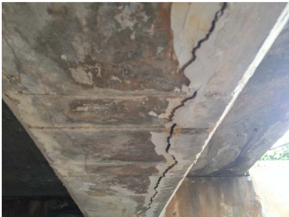
Figure 24: Beam Cracking Island Drive Structure
