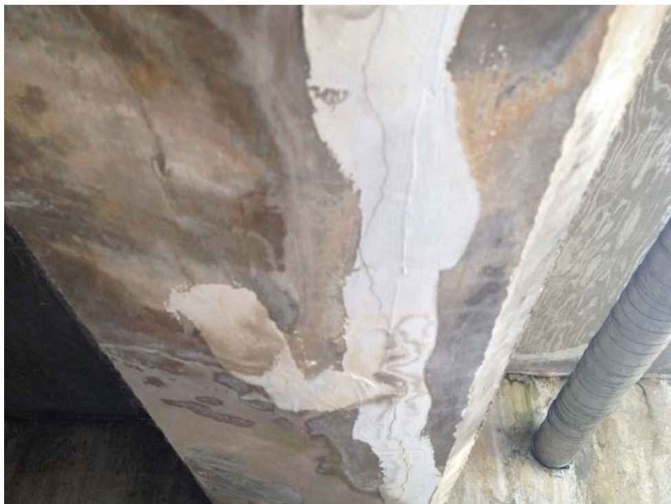
Figure 20: Beam Cracking Island Drive Structure
