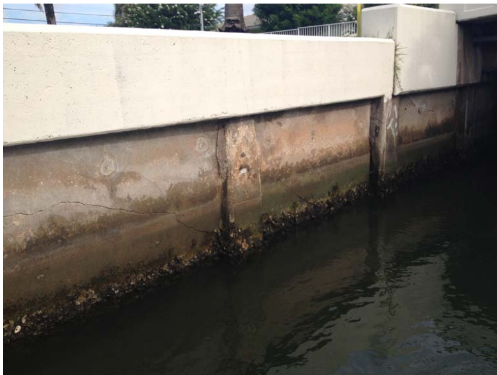
Figure 36: Sheet Panel Cracking Island Drive Structures
