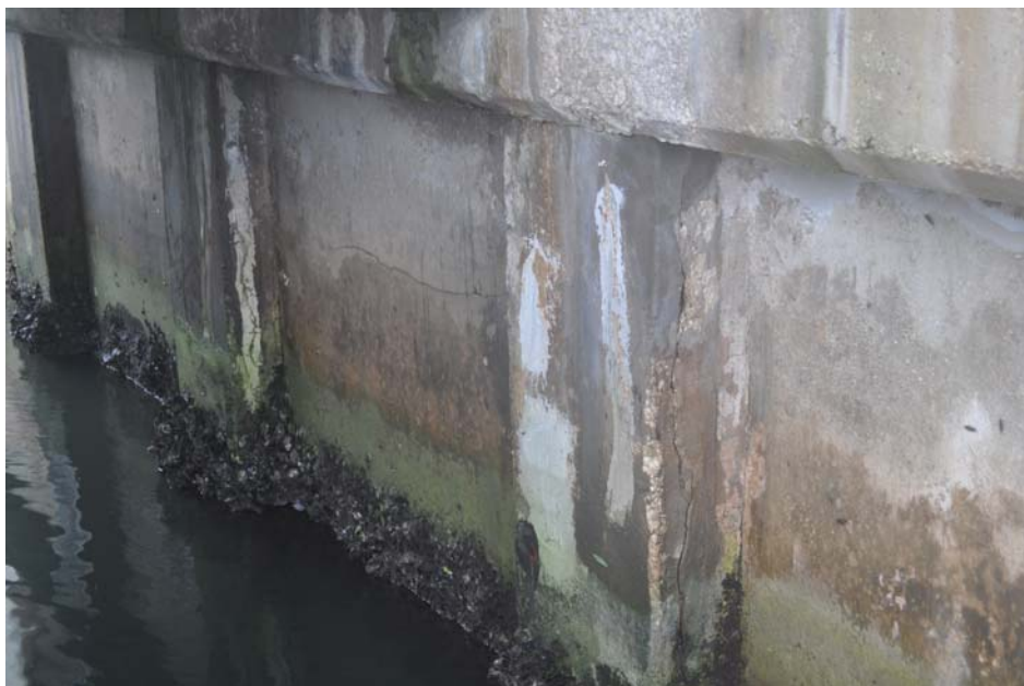
Figure 12: Pile Cracking Island Drive Structure
