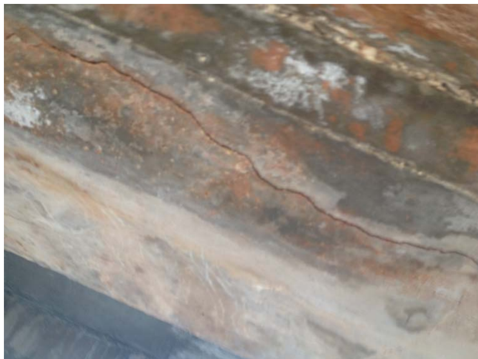
Figure 19: Beam Cracking Island Drive Structure
