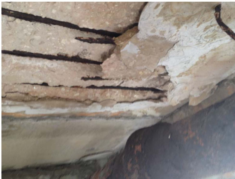
Figure 40: Deck Spalling & Reinforcing Corrosion Grand Bahama Lane Structure
