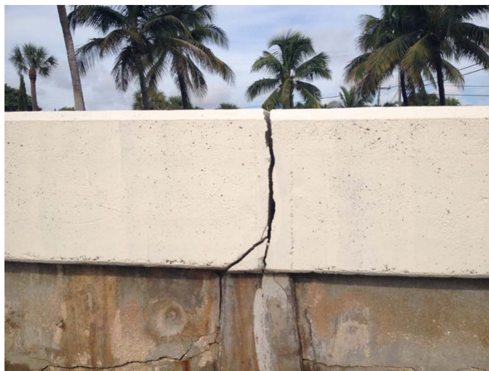
Figure 35: Bulkhead Cap Cracking Island Drive Structures
