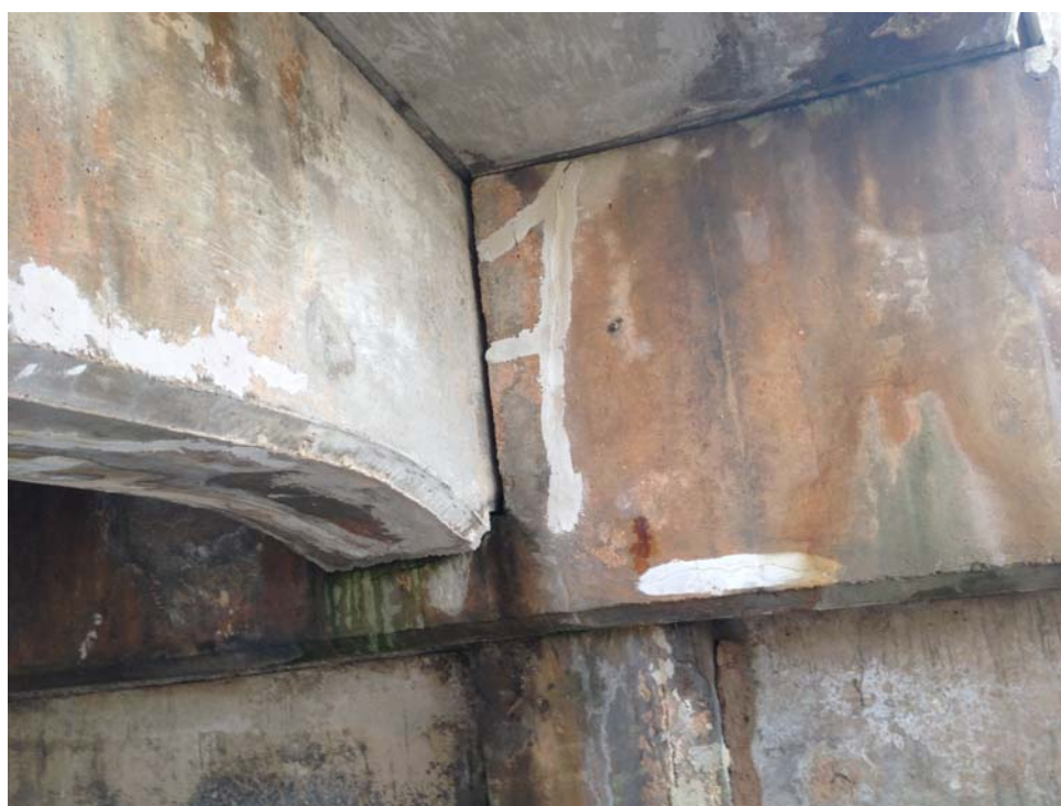
Figure 15: Cap Cracks Island Drive Structure
