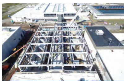
New chemical building with ancillary systems
