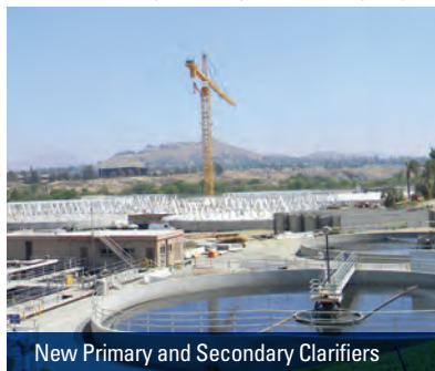
Primary Clarifiers during cover installation
