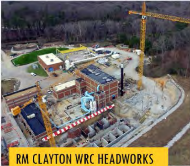
RM CLAYTON WRC HEADWORKS IMPROVEMENTS DESIGN-BUILD
