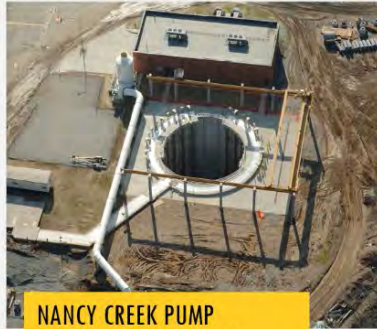
NANCY CREEK PUMP STATION DESIGN-BUILD
