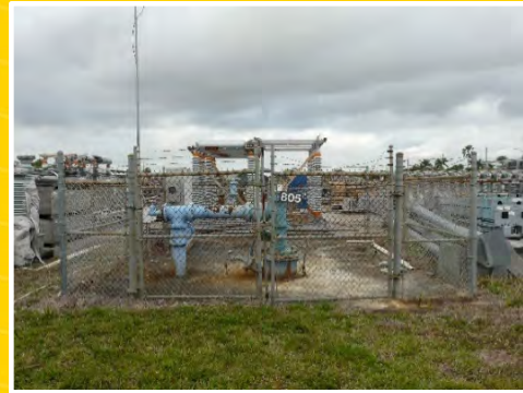
Exhibit 3-6 / Well 805 prior to well rehabilitation
