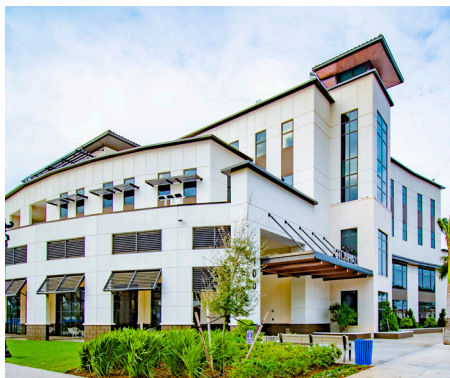
Boynton Beach City Hall, Library and District Energy Plant City of Boynton Beach
