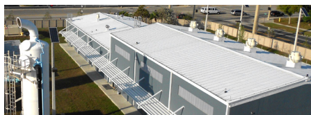
Nanofiltration WTP City of Dania Beach
