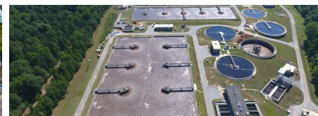
Lower Poplar and Rocky Creek WRF Upgrades Macon Water Authority
