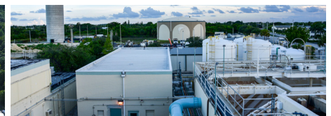
Boynton Beach WTP Improvements City of Boynton Beach
