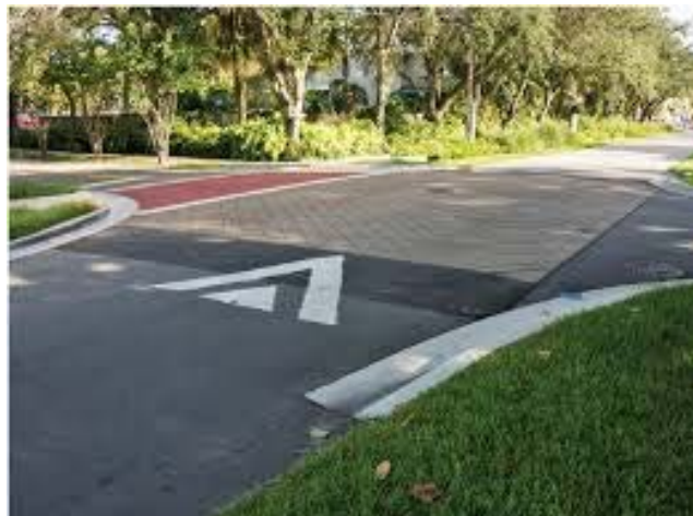
Figure 4.3.a: Raised Intersection Example
