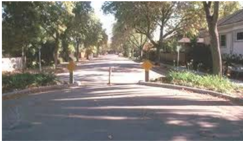
Figure 4.7.a: Permanent Road Closure Example
