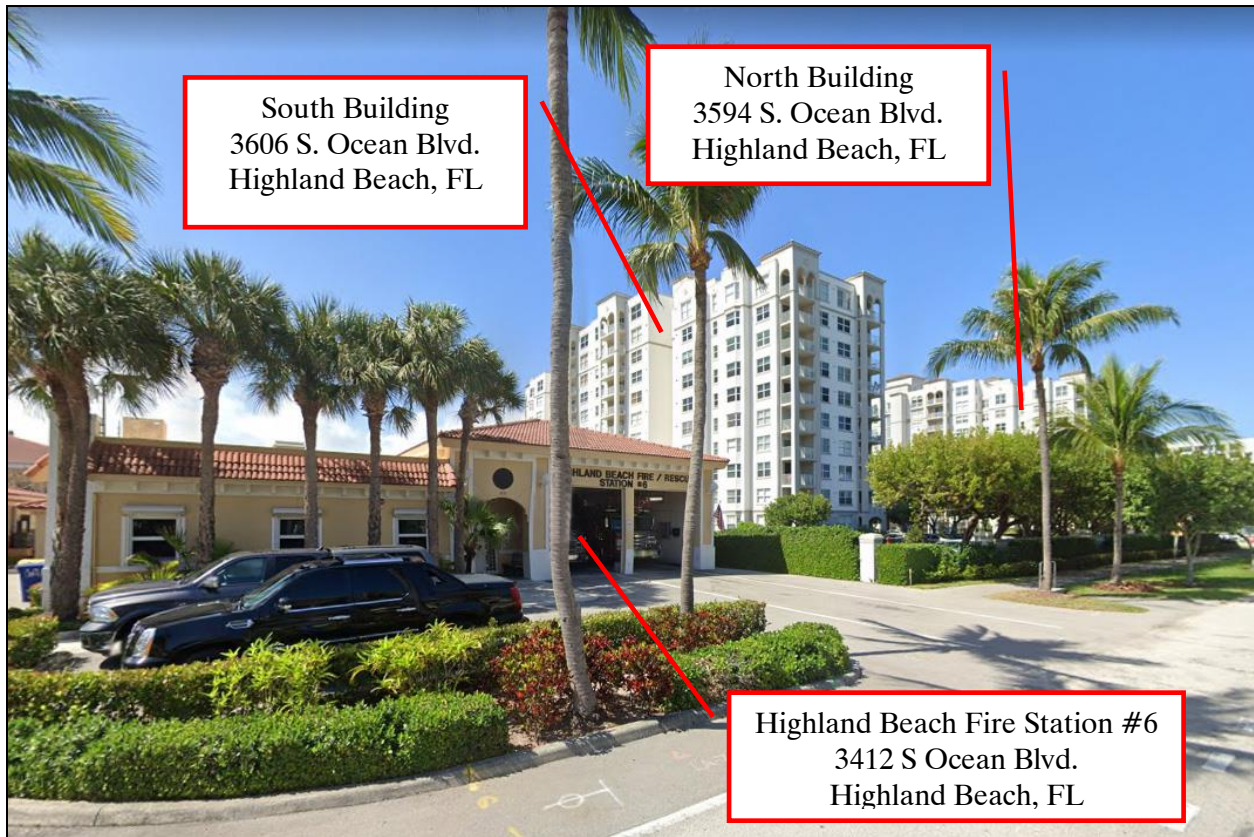
Front View of Fire Station #6 with Highland Beach Club Condominiums in background, looking NW
