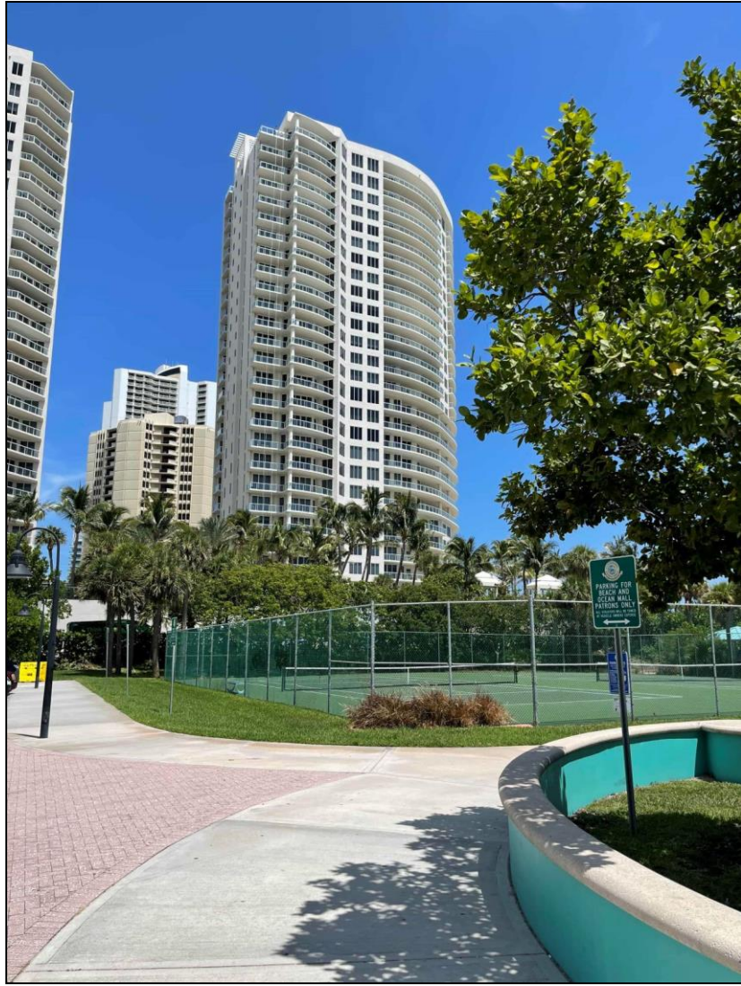
View of The Ritz Carlton Residences – Tower 1 Looking Northeast from Ocean Avenue at Walkway to Tennis Courts
