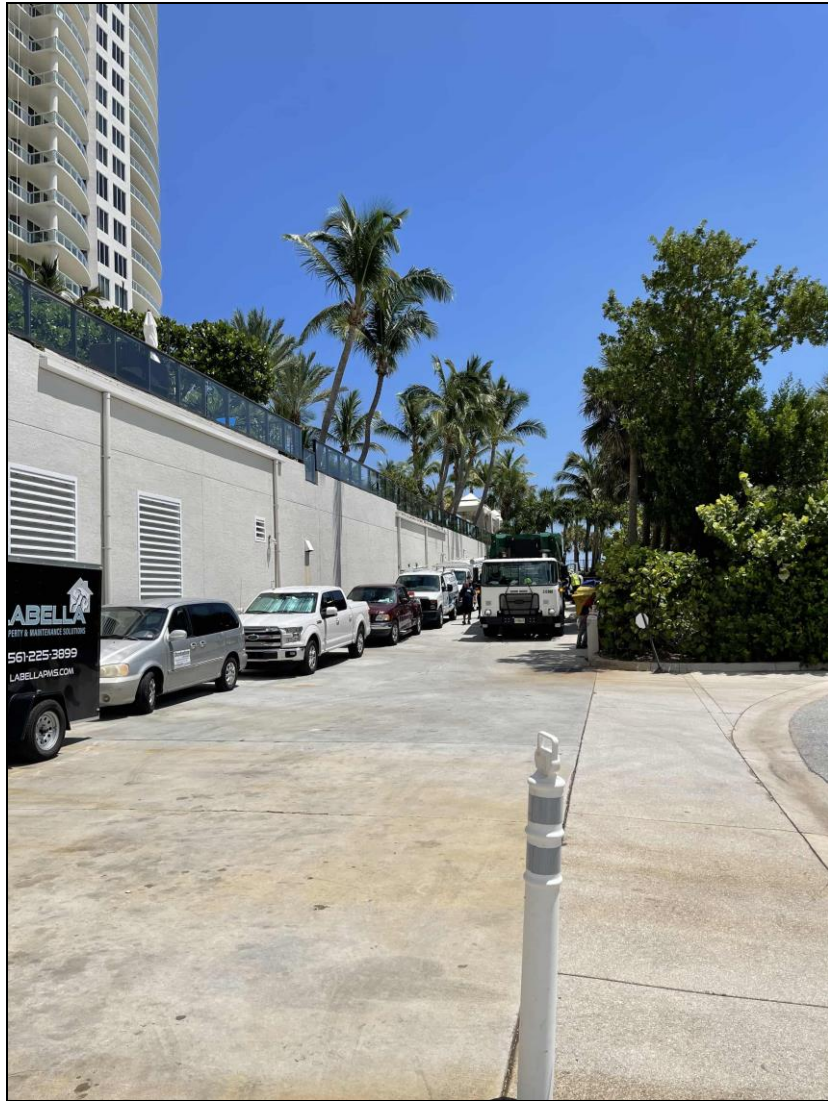
View of The Ritz Carlton Residences – Service Alley Looking East from Ocean Avenue Along the Southern Property Line
