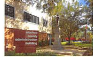
Industrial / Office Park Development / Construction
