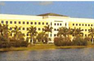
160,000 sf Office Building Development / Construction
