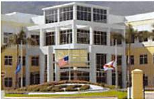
300,000 sf Office Building Development / Construction
