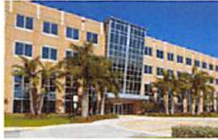
Industrial / Office Park Development / Construction
