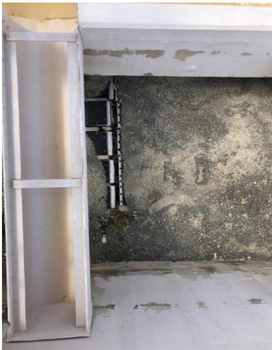
Figure 4-4. Failed Underdrain Emerged Through Media Surface
