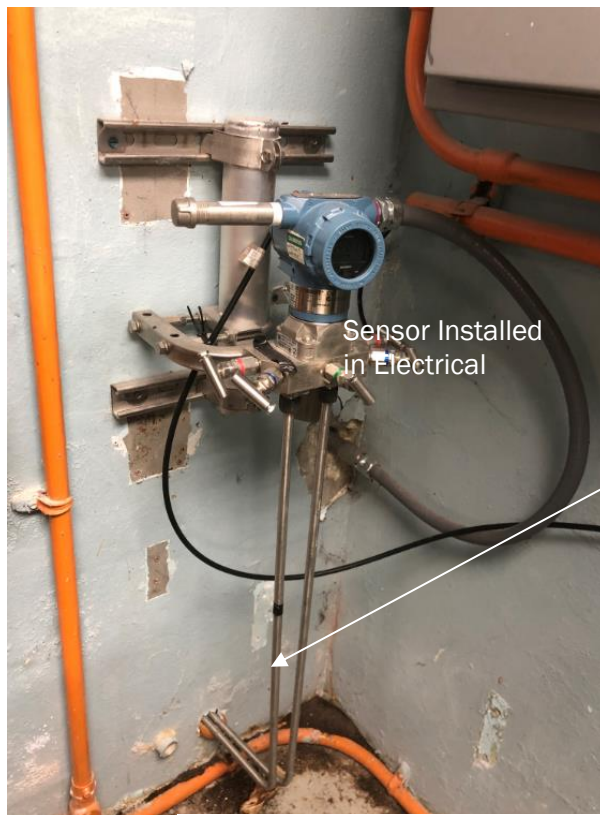
Figure 4-9 and Figure 4-10. Arrangement of Venturi Meter and Sensor Lines
