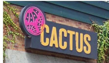
Figure 46 Cabinet sign with push through or routed copy
