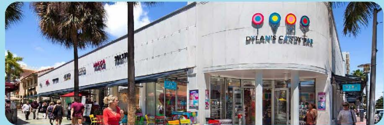
Figure 41 Image of building in Coconut Grove in Miami from Visitors Bureau with multiple tenants and consistent awnings, lighting and letter size. Each tenant uses their own logo or font to create identity but conforms to the standards of the building.
