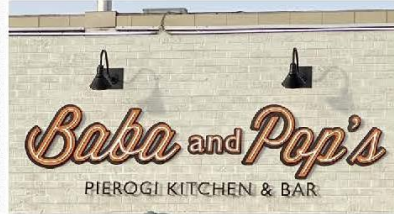
Figure 43 Reverse illuminated channel letters on concealed raceway
