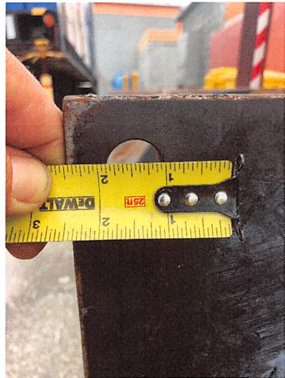
Figure 5. Sole plate bolt holes of uninstalled pumps
