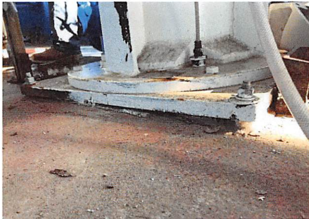
Figure 4. Caulk under sole plate of HSP No. 6
