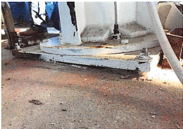
Figure 4. Caulk under sole plate of HSP No. 6
