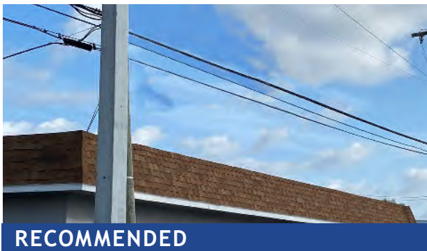
Figure 3 After image with nonconforming sign removed.
