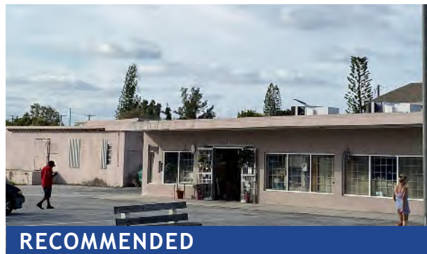
Figure 5 After image with nonconforming sign removed.
