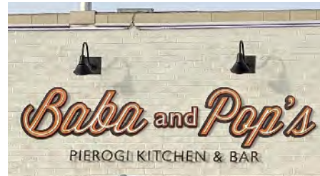
Figure 43 Reverse illuminated channel letters on concealed raceway
