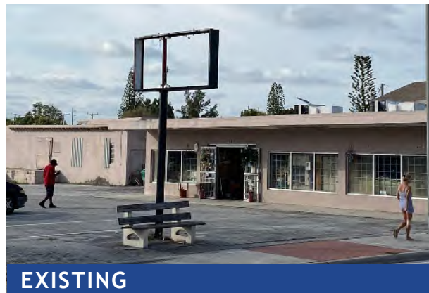
Figure 4 Image of empty sign which does not meet existing code.
