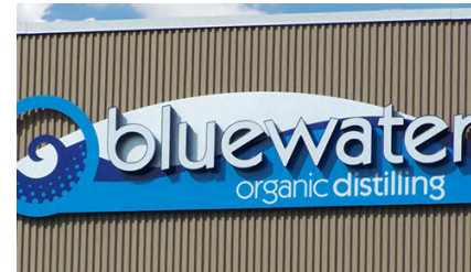
Figure 44 Face illuminated channel letters mounted on wireway
