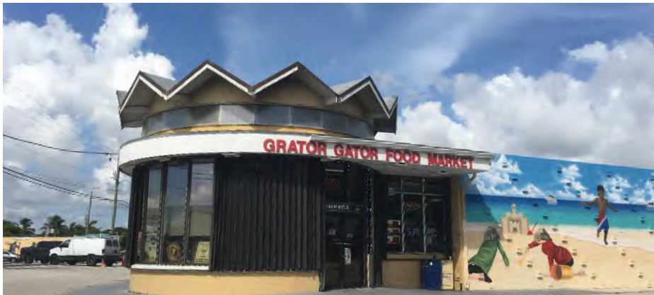
Figure 8 The unique roof profile of historical architectural style.
