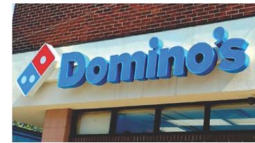
Figure 5 Face illuminated channel letters mounted on raceway
