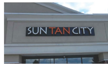
Figure 4 Face illuminated channel letters mounted on wireway
