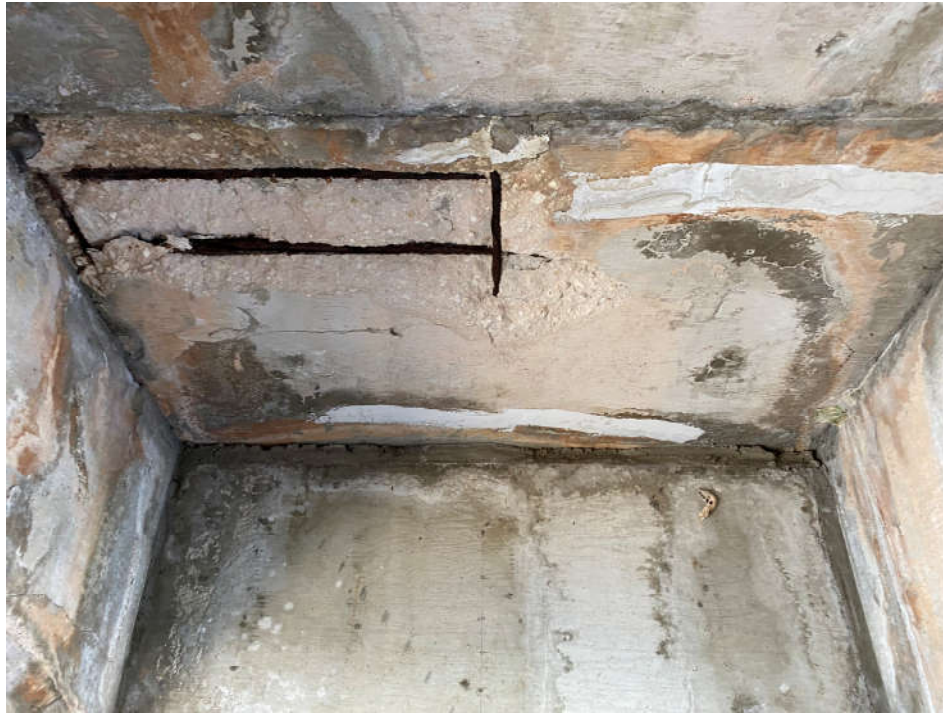
Photo 5: Grand Bahama Lane – West Bridge Underside of Deck
