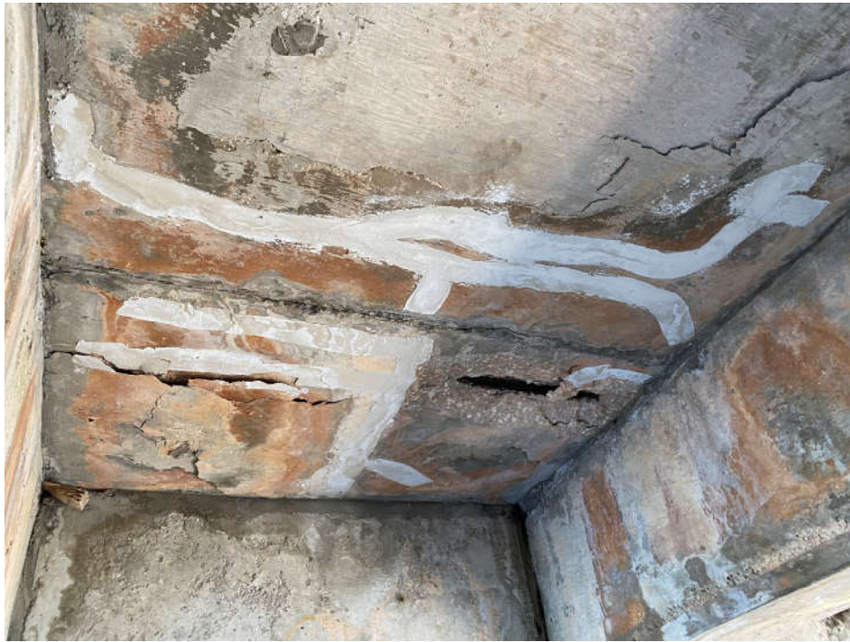
Photo 3: Grand Bahama Lane – East Bridge Underside of Deck
