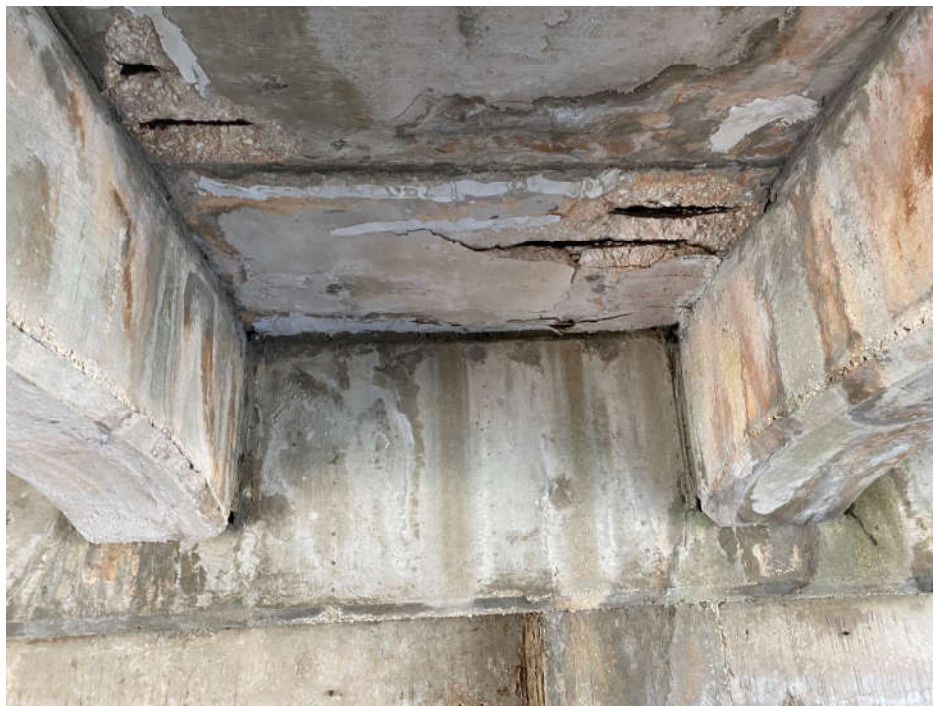
Photo 6: Grand Bahama Lane – West Bridge Underside of Deck
