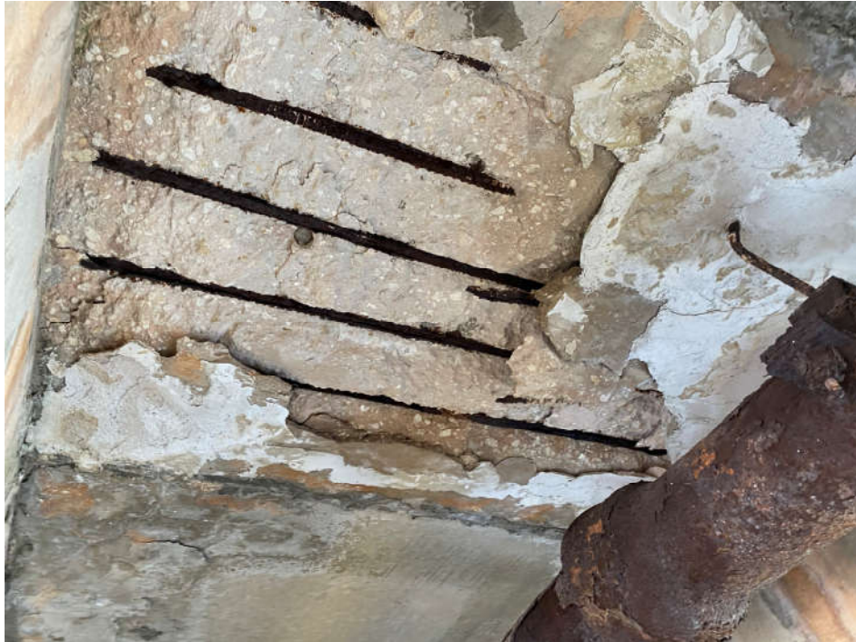
Photo 7: Grand Bahama Lane – West Bridge Underside of Deck
