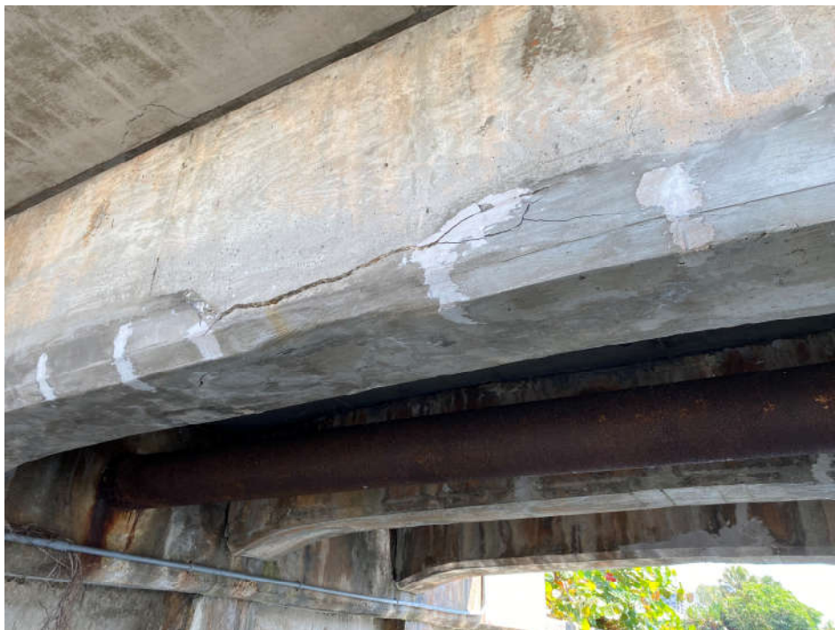
Photo 17: Island Drive – SE Bridge Outer Beam North Side
