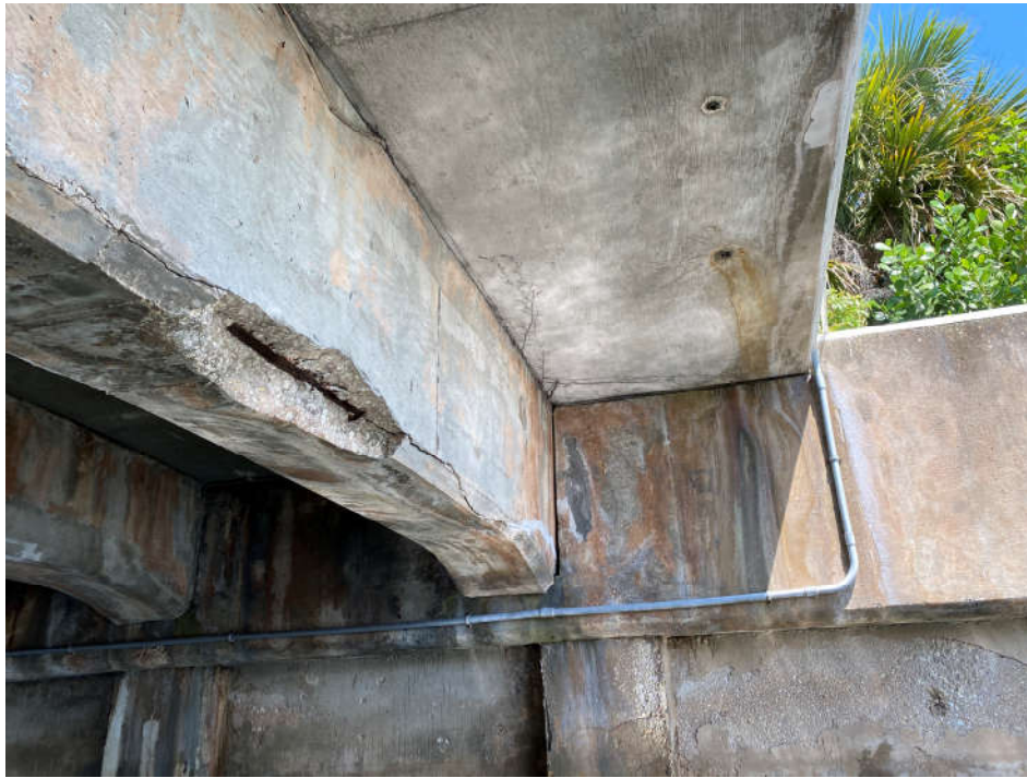
Photo 15: Island Drive – SE Bridge Outer Beam South Side
