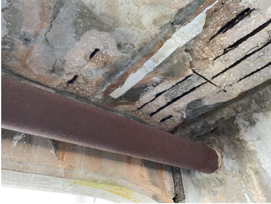
Photo 1: Grand Bahama Lane – East Bridge Underside of Deck
