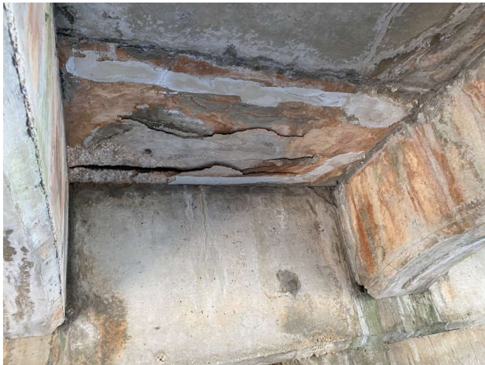
Photo 4: Grand Bahama Lane – East Bridge Underside of Deck
