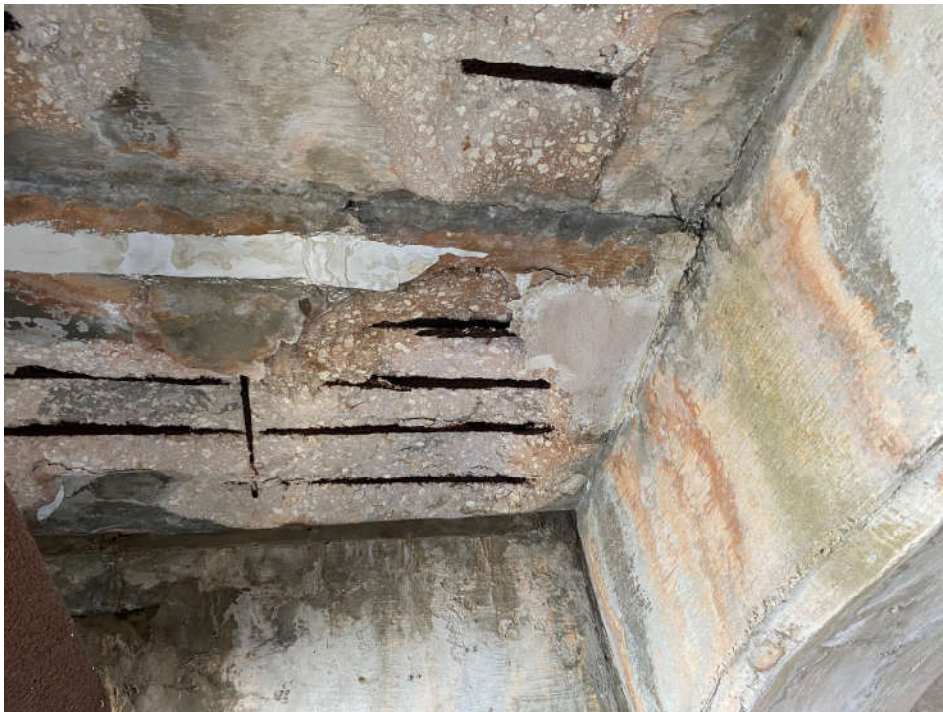
Photo 2: Grand Bahama Lane – East Bridge Underside of Deck
