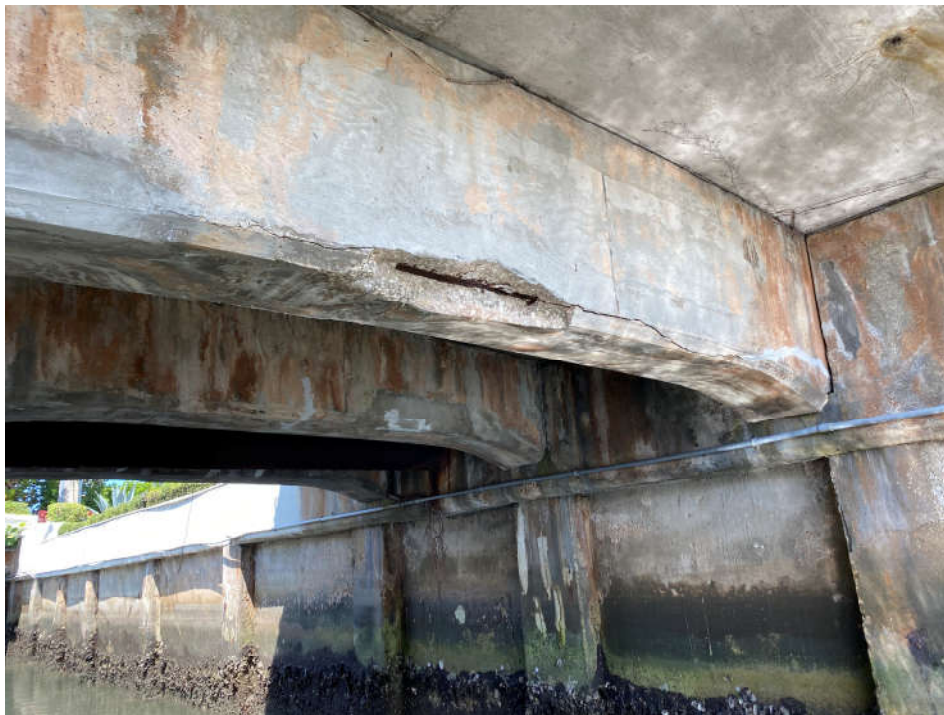
Photo 16: Island Drive – SE Bridge Outer Beam South Side
