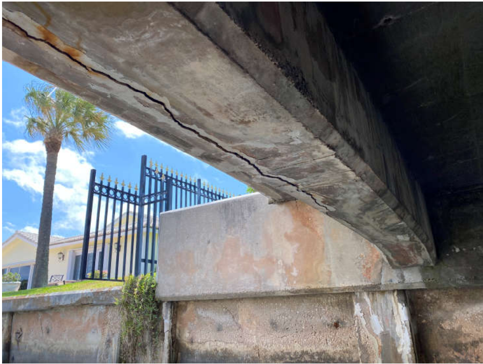
Photo 14: Island Drive – SW Bridge Outer Beam South Side
