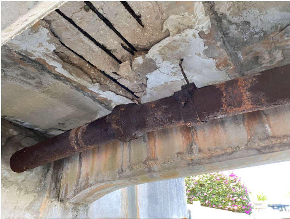
Photo 8: Grand Bahama Lane – West Bridge Underside of Deck
