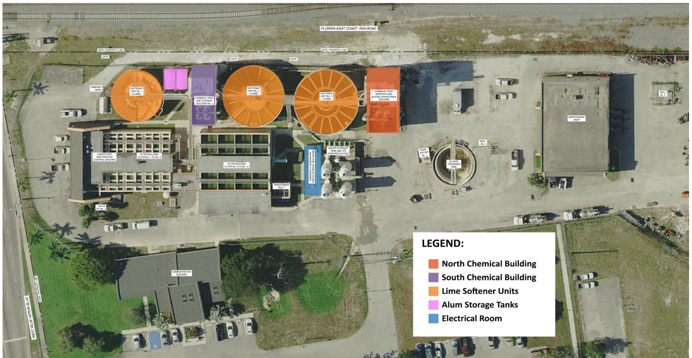
RIVIERA BEACH WTP - AERIAL VIEW
