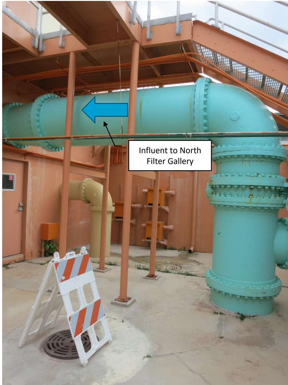
Figure A-7. Influent pipe (south side) of North Filter Gallery
