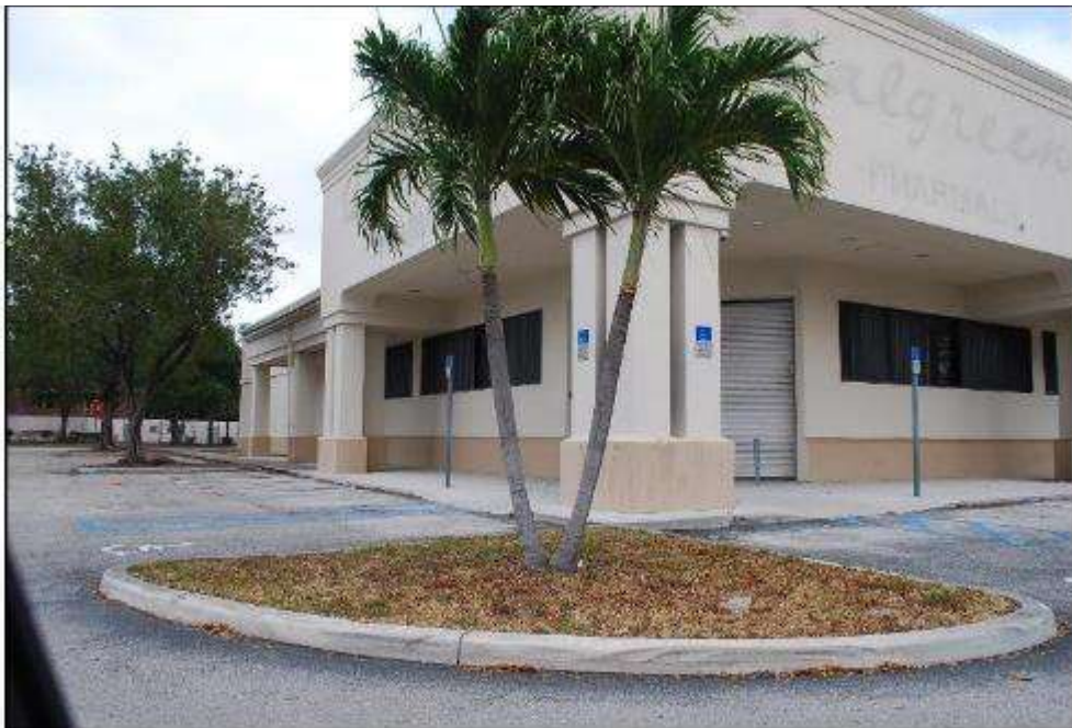
West side of Walgreen's building, looking north
