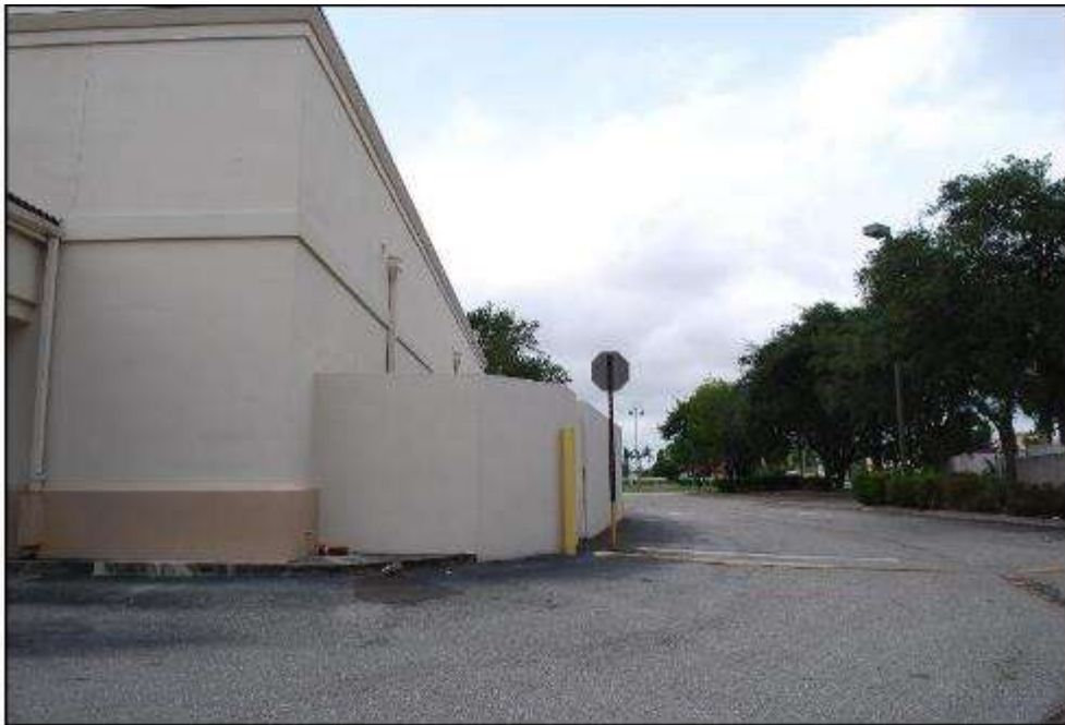
North side of property, looking west
