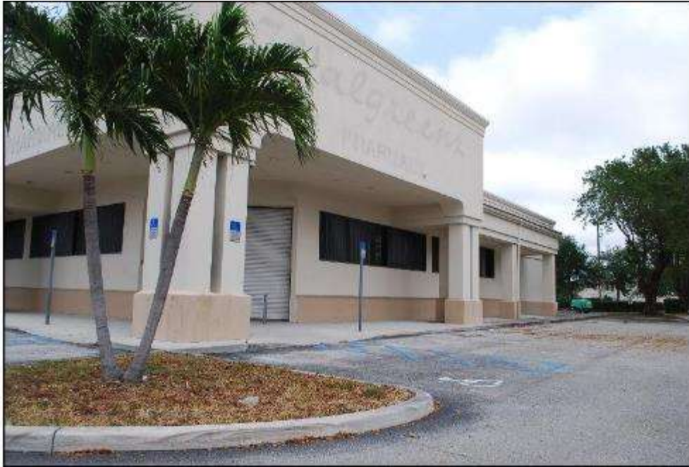
South side of Walgreen's building, looking northeast
