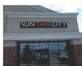
FACE ILLUMINATED CHANNEL LETTERS MOUNTED ON WIREWAY
