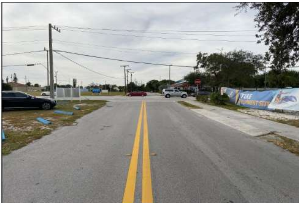
East 12 th Street facing east
