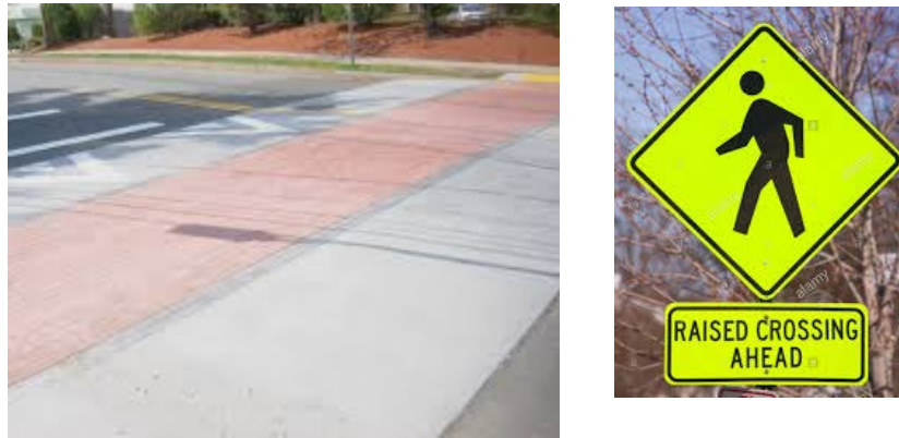
Figure 4.4.a: Raised Crosswalk Example
