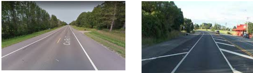
Figure 4.1.a: Narrowing Lanes Striping Examples
