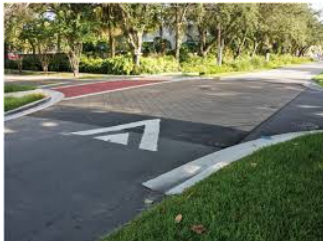
Figure 4.3.a: Raised Intersection Example
