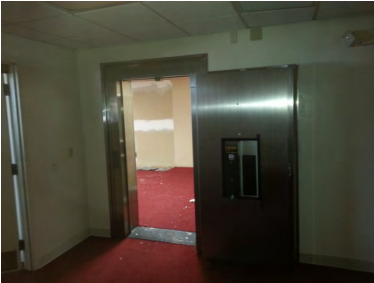
79. View in the entry door into the bank vault noted in the southwest portion of the 1 st floor.
