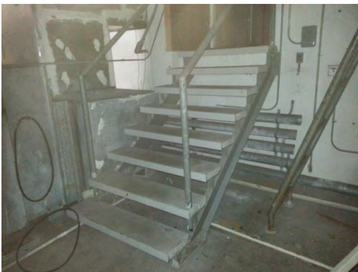
90. View of the access stair noted in the mechanical room in the west portion of the building.
