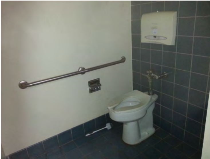
67. View in the 1 st floor men's toilet room noting the handicapped accessible water closet stall.
