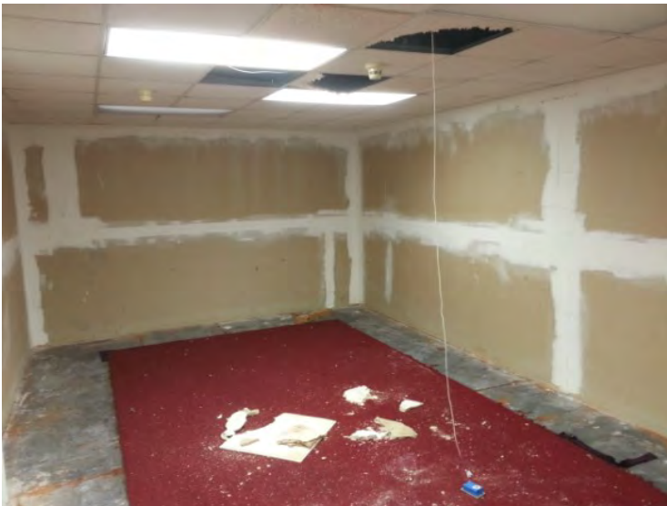
80. View in the bank vault noted in the southwest portion of the 1 st floor.
