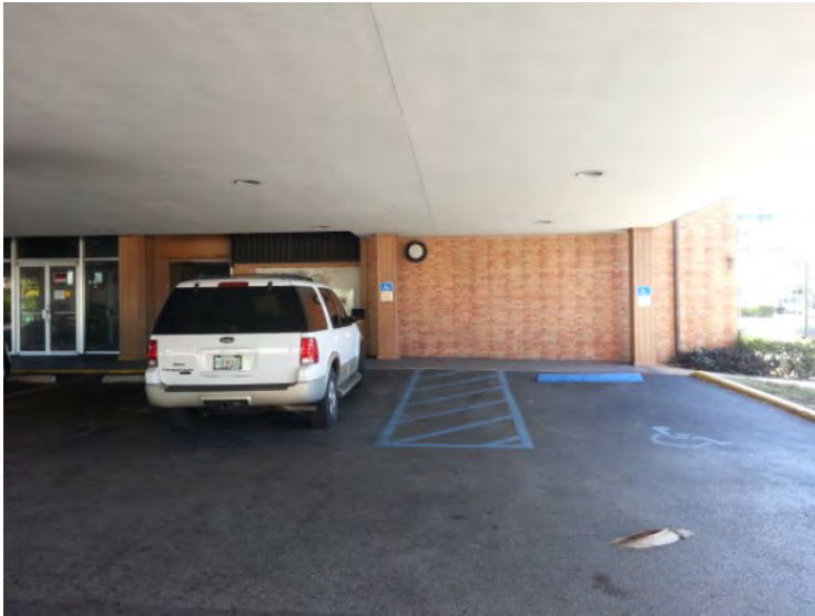
40. View of handicapped accessible parking spaces provided at the carport.
