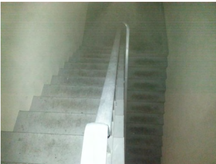
63. View of the northwest stairway.
