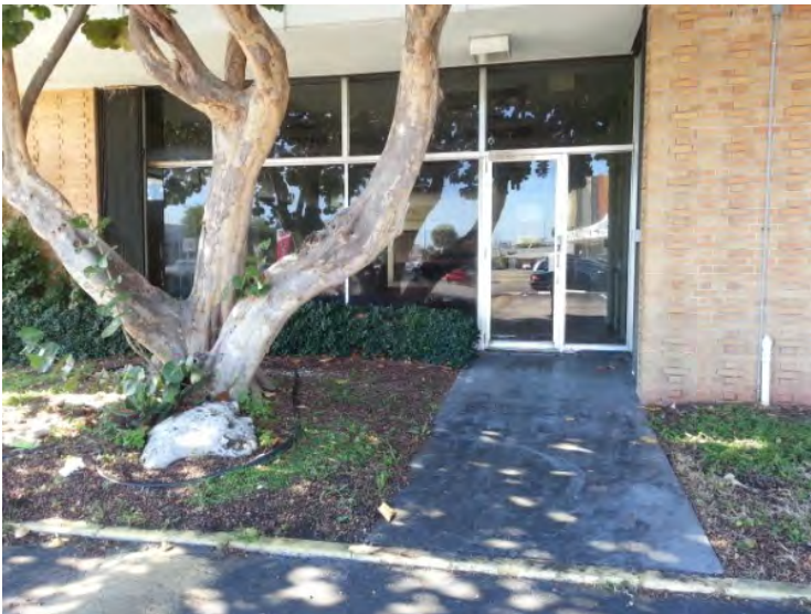
50. View of the east entry door to the building.
