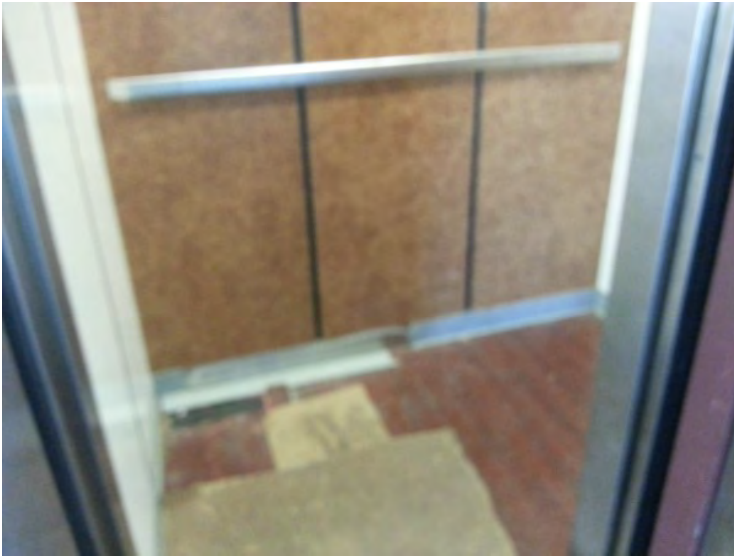
58. View in the elevator noting the floor and wall finishes.
