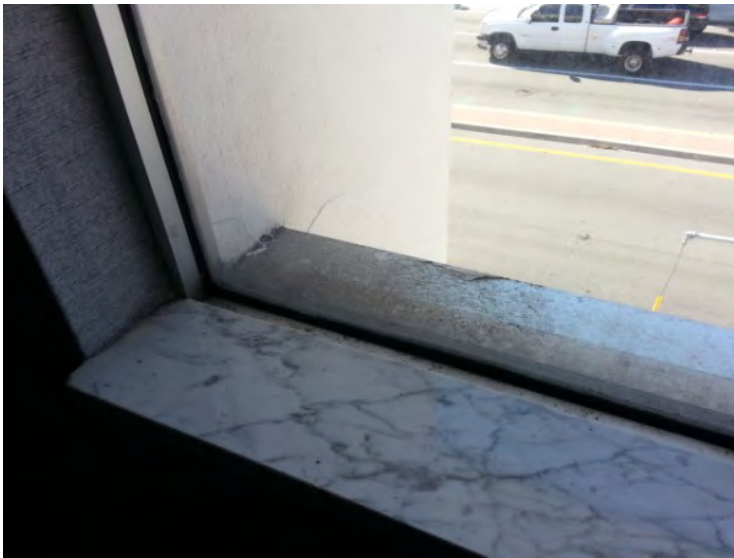
73. View of typical interior window sill.
