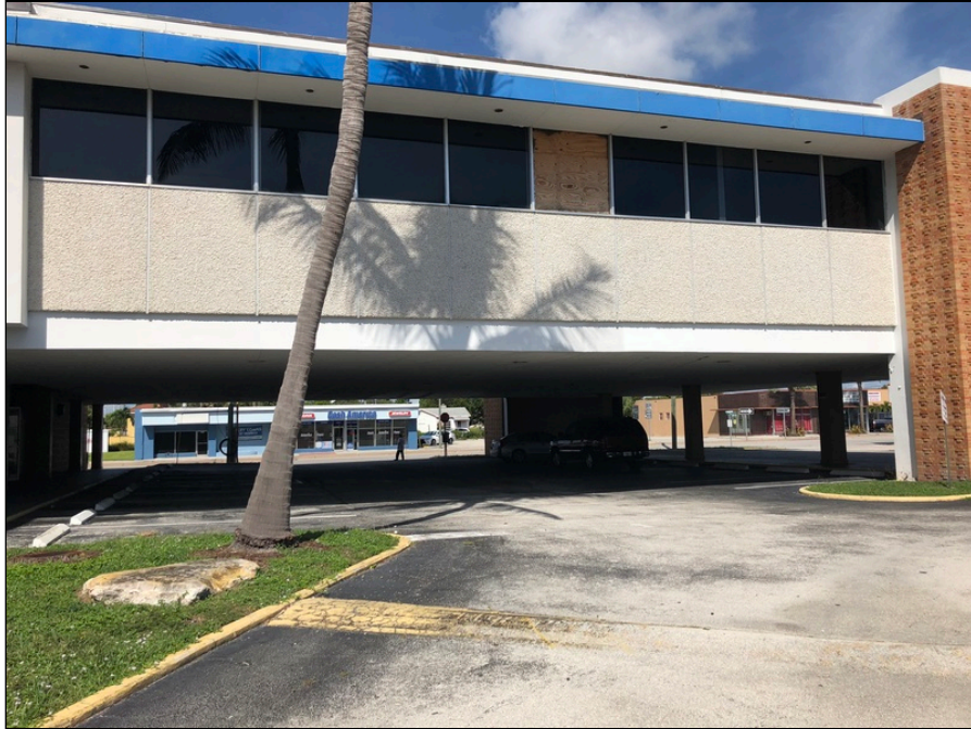
11 - View of raised second floor from east looking west
