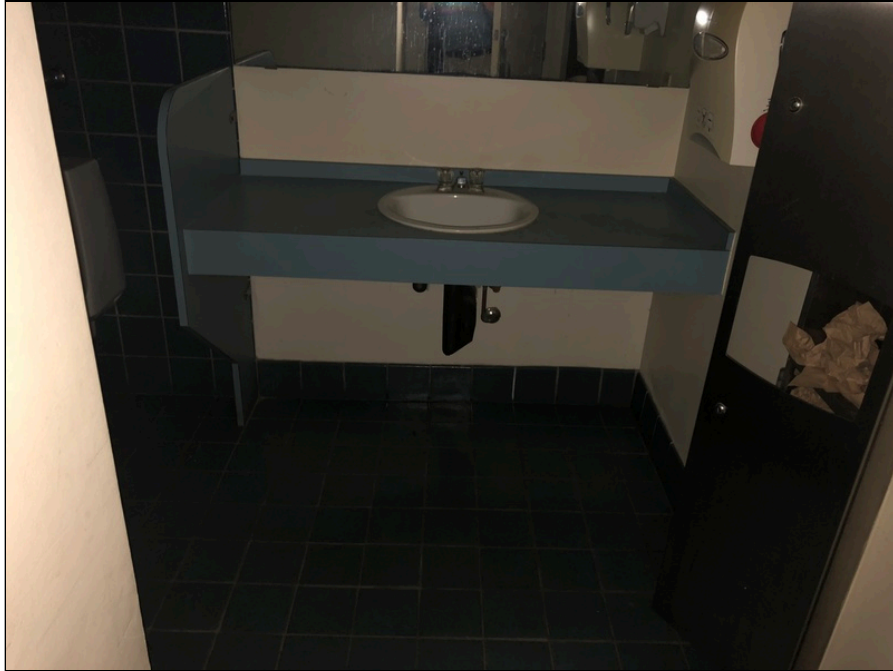
7 - One of the building restrooms
