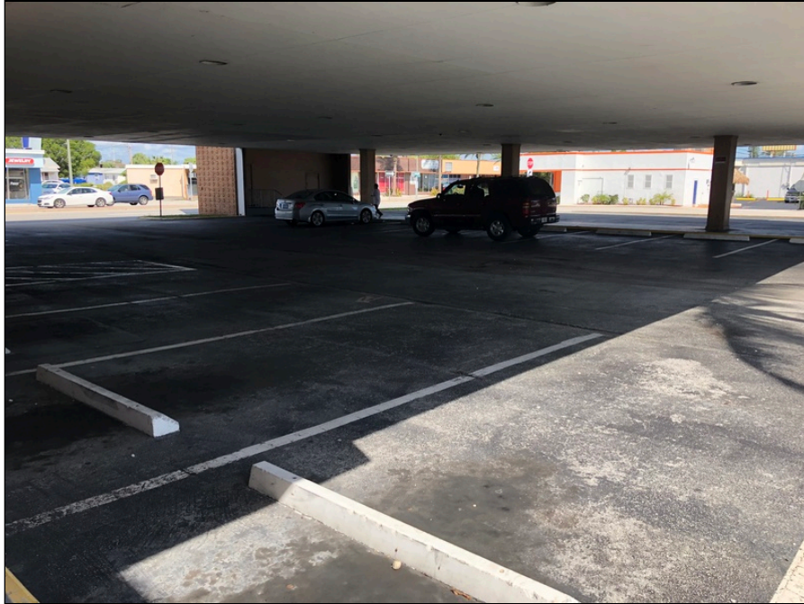
13 - Covered parking area beneath raised second floor of building
