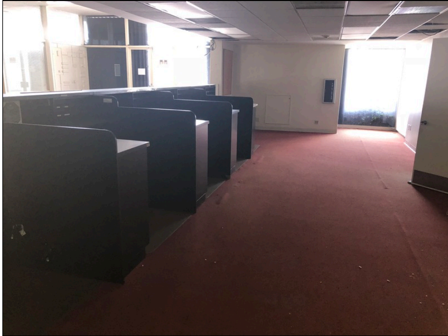
3 - Former bank teller area on main level
