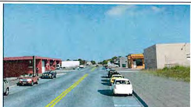
Phase 1: To enhance retail and calm traffic, on-street parking, curb, gutter, and sidewalks are added.
