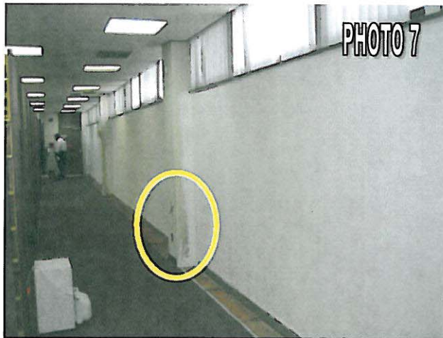
Library south wall – Drywall on column with SVM.
