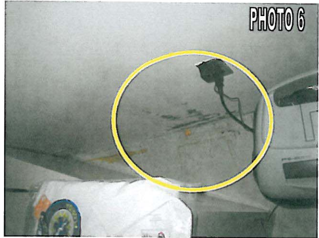
Fire Department Room F03 – SVM on west wall at baseboard.
