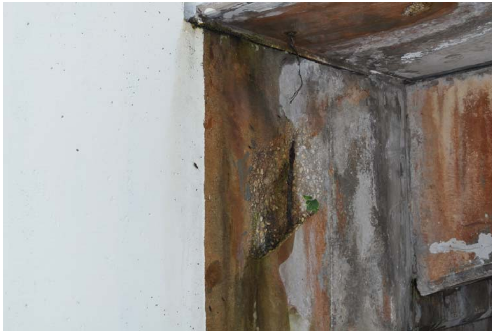
Figure 14: Cap Spall Island Drive Structure
