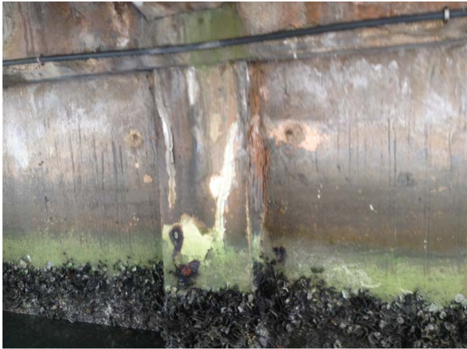
Figure 10: Substructure Island Drive
