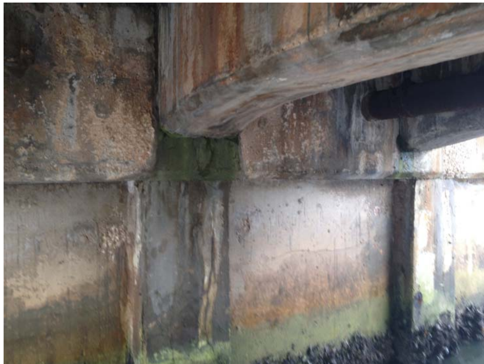
Figure 11: Substructure Island Drive
