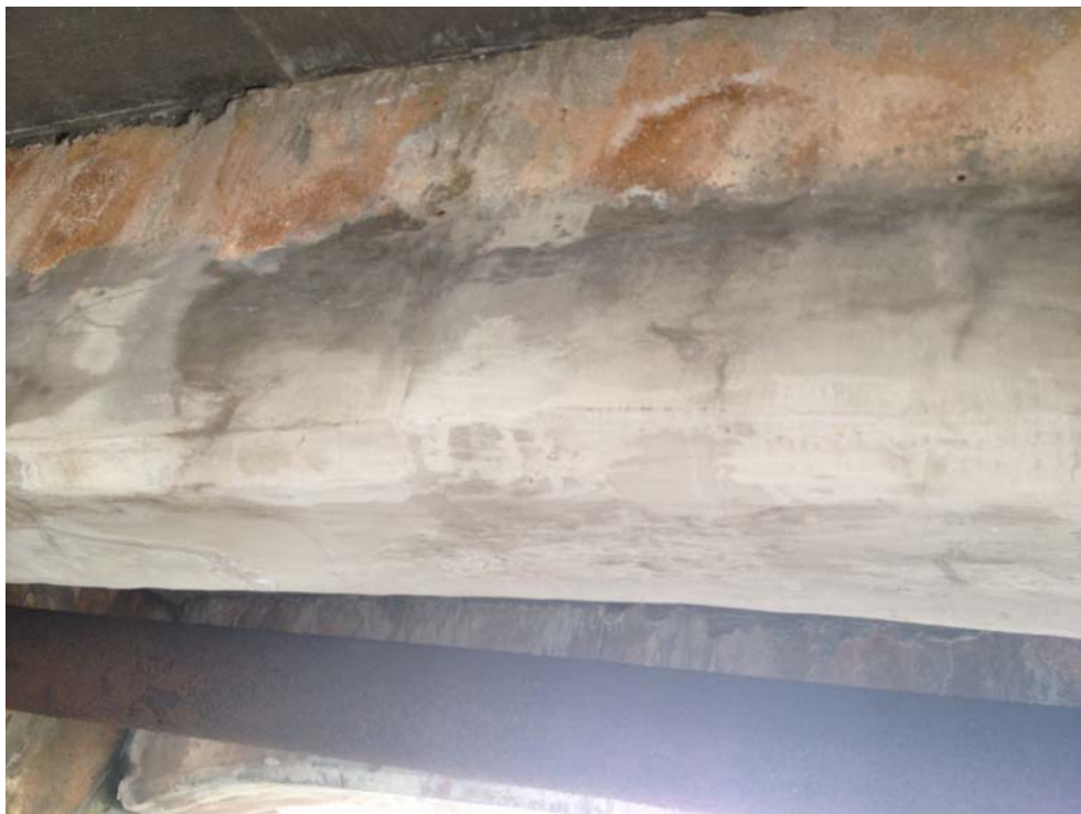
Figure 31: Beam Repair Island Drive Structure
