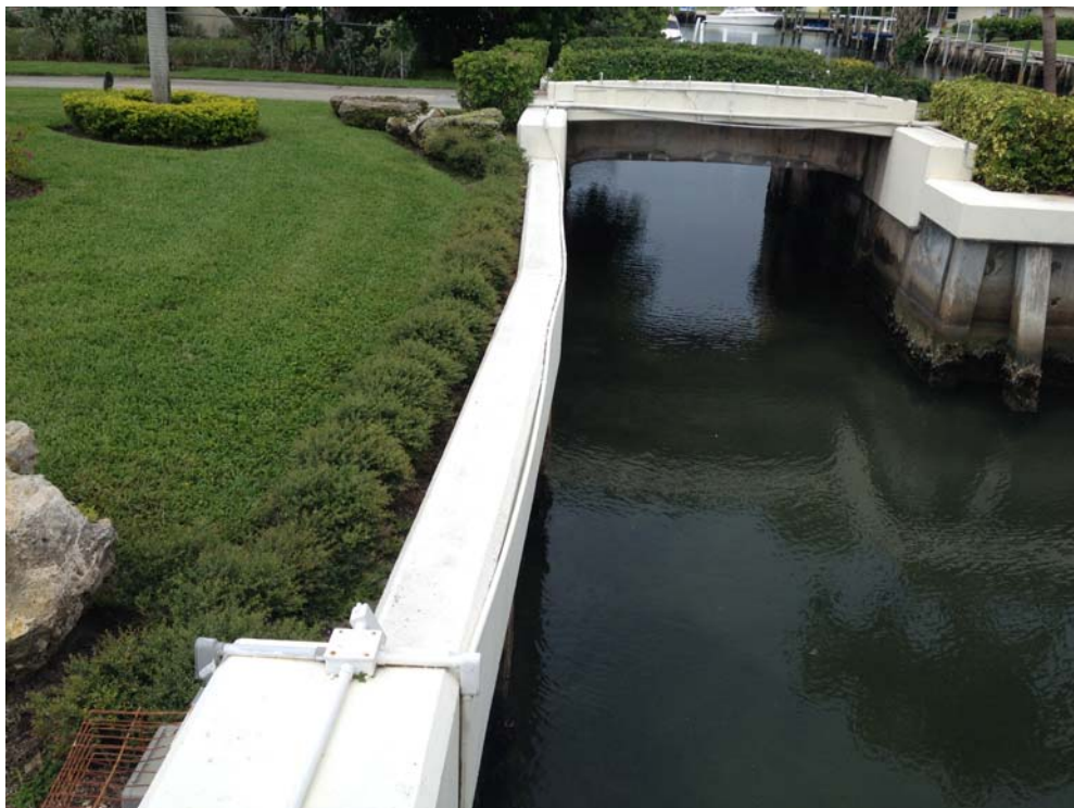
Figure 33: Bulkhead Wall Deflection Island Drive Structures
