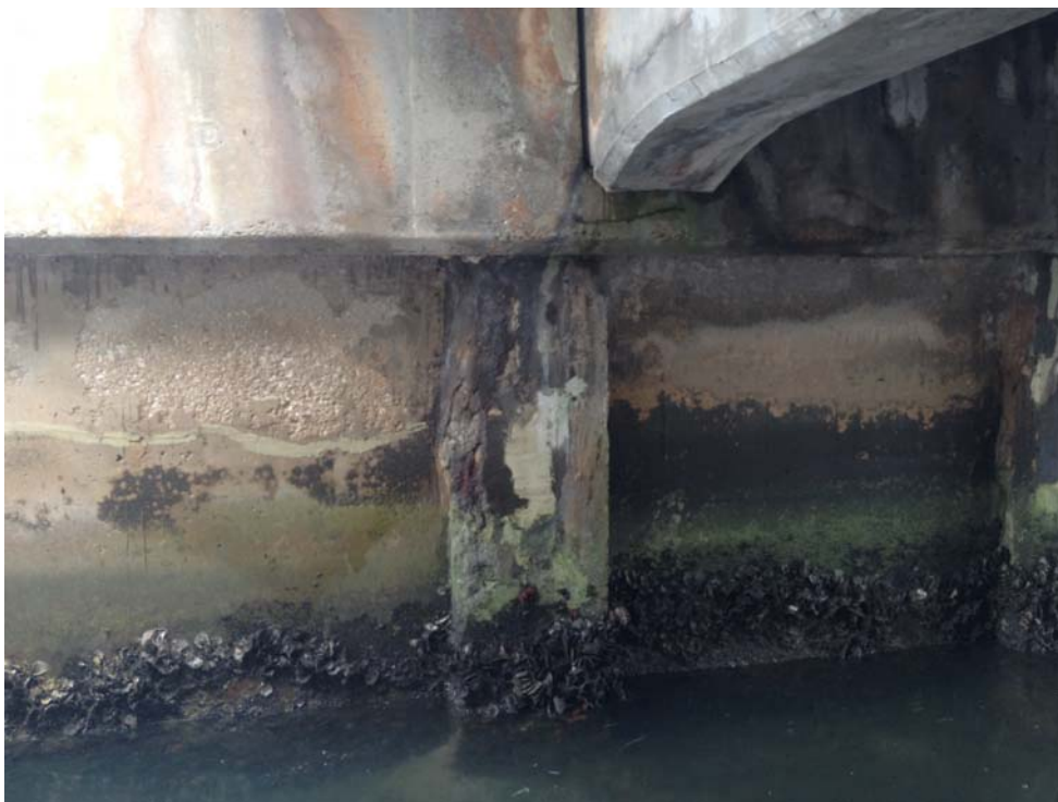
Figure 9: Substructure Island Drive
