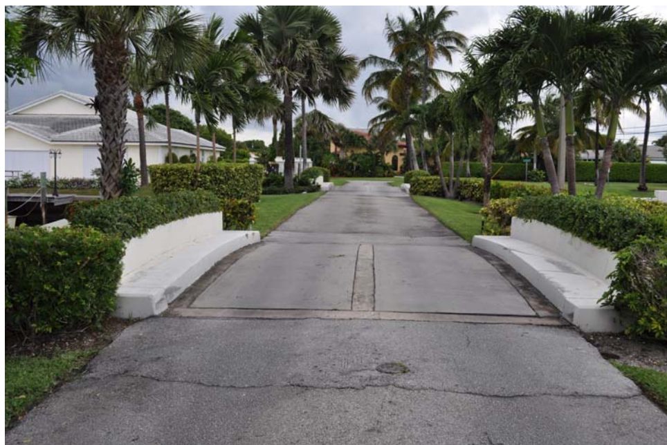
Figure 5: Structure at Island Drive
