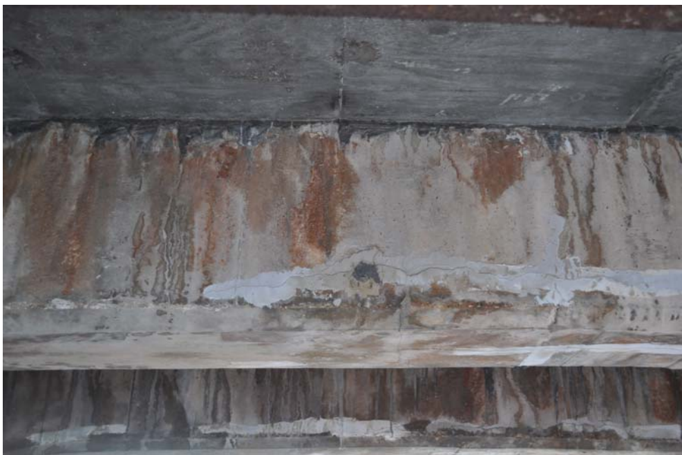
Figure 17: Deck Slab & Beam Island Drive Structure
