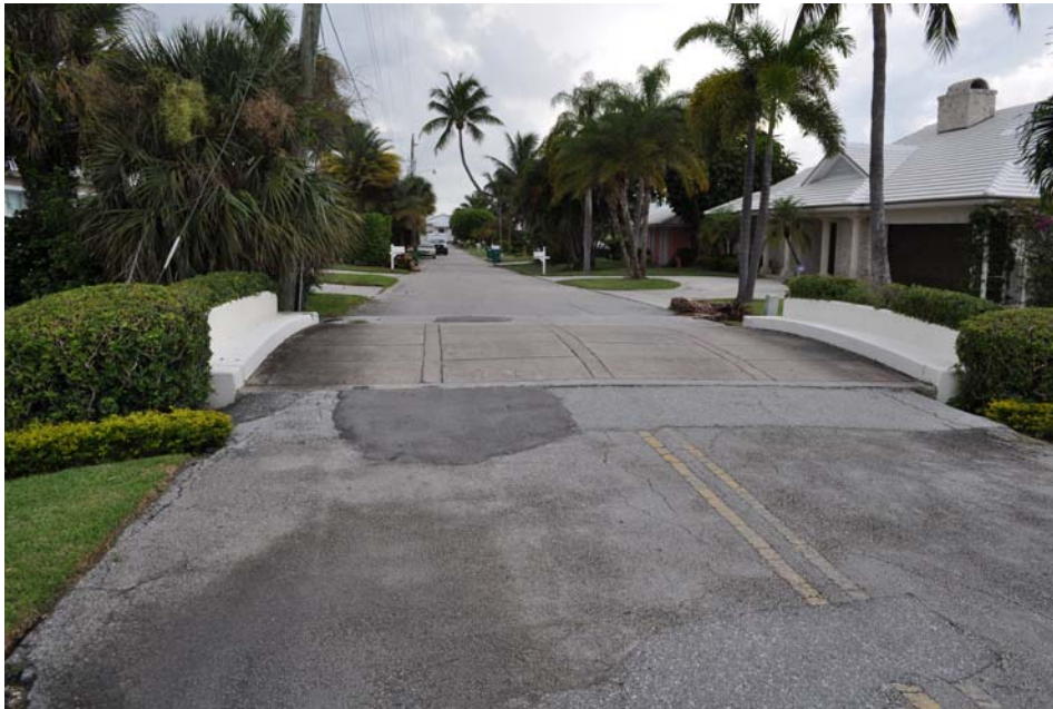
Figure 7: Structure at Grand Bahama Lane
