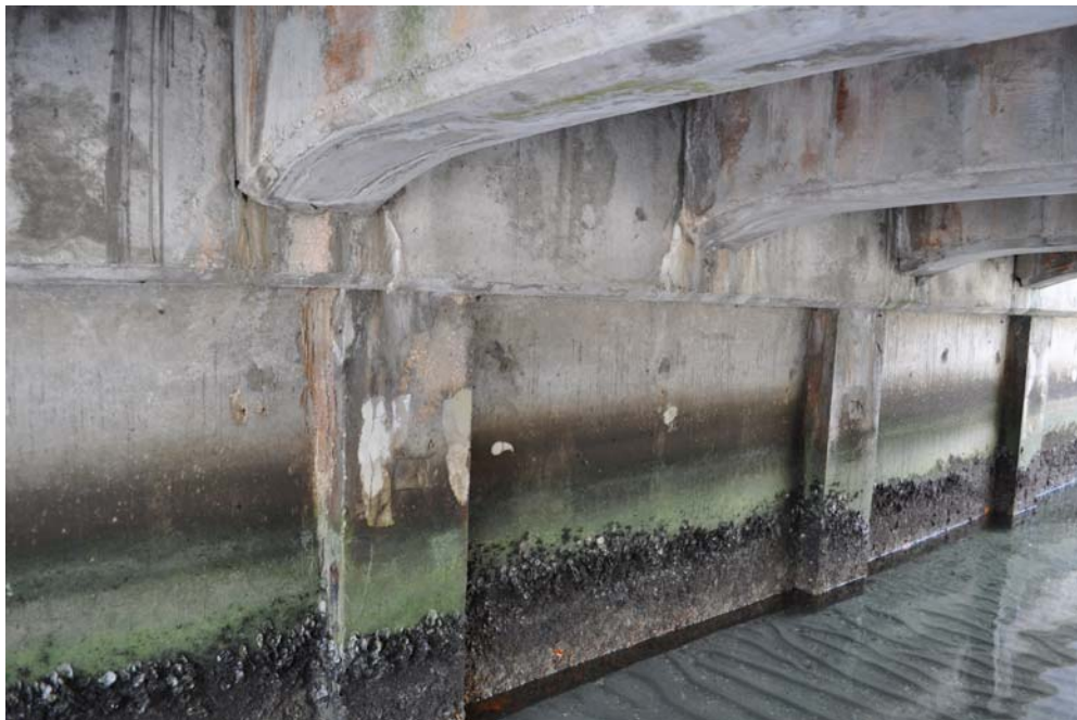
Figure 37: Substructure & Deck Beams Grand Bahama Lane Structure
