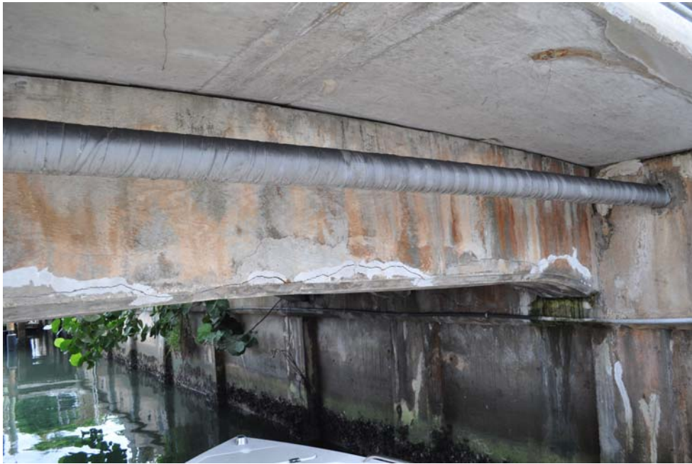
Figure 18: Deck Slab & Beam Island Drive Structure
