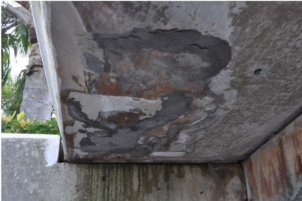
Figure 16: Slab Under Planter Island Drive Structure
