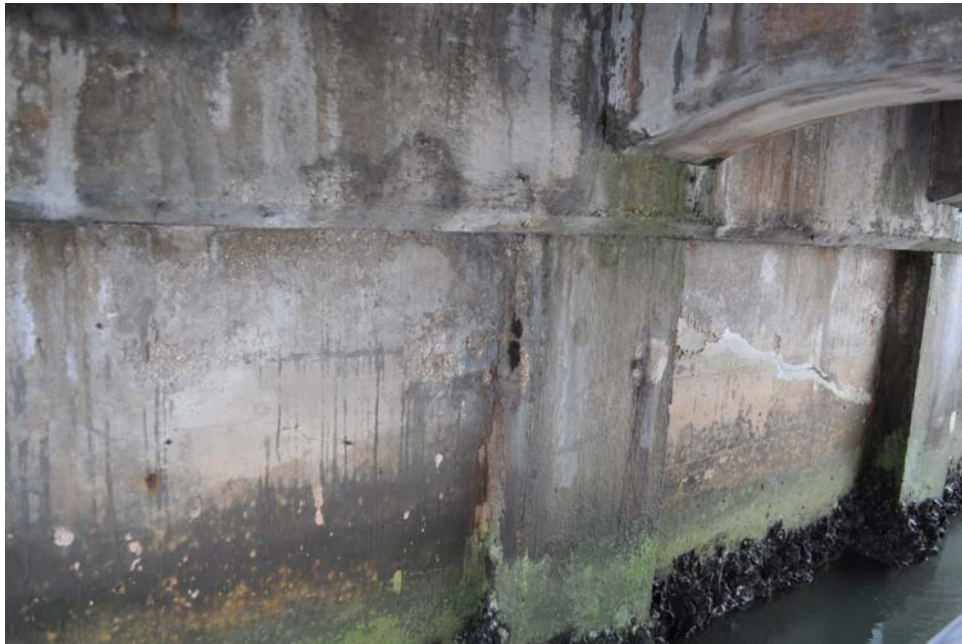
Figure 8: Substructure Island Drive
