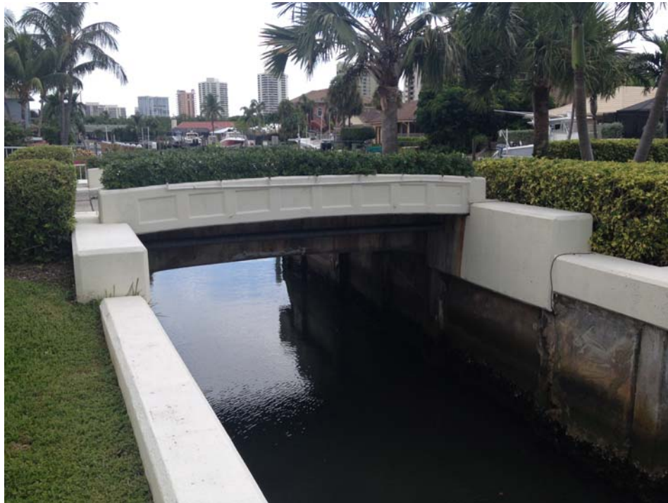
Figure 4: Structure at Island Drive
